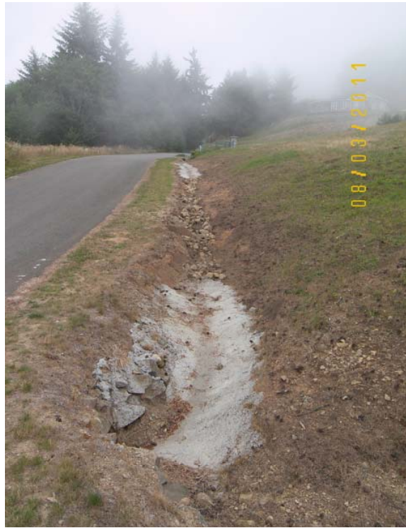
Figure 4: This drainage ditch along one of the roads in the Major Hillside Subdivision had eroded and incised, creating a potential for plugging the ditch relief culvert. There had been attempts to stop the incision by installing concrete in some locations.
