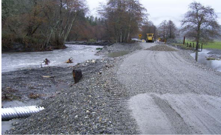
Figure 18: Bar Road at the completion of emergency road repair. Note the barren condition of the stream bank.
