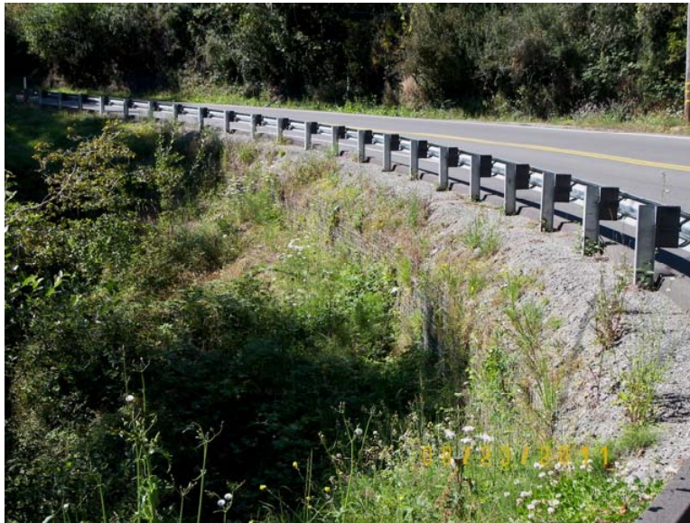
Figure 25: This gabion wall was installed at stream crossing on Scenic Drive to reduce likelihood of slope failure.
