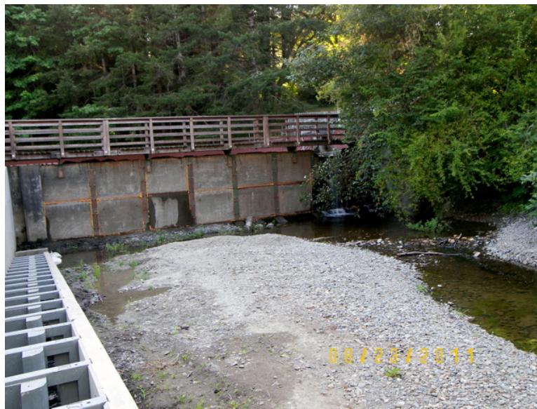
Figure 21: Seasonal dam on Freshwater Creek. The entire structure is installed every year in June and removed in late August. The fish ladder is on the left of the picture. The side channel connecting the ladder to the main channel is at the base of the dam.
