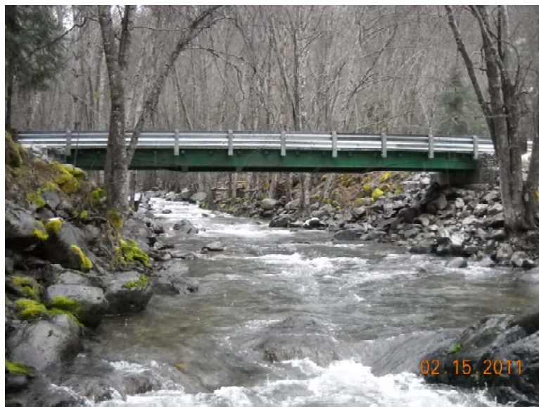
Figure 10: The new Canyon Creek Bridge
