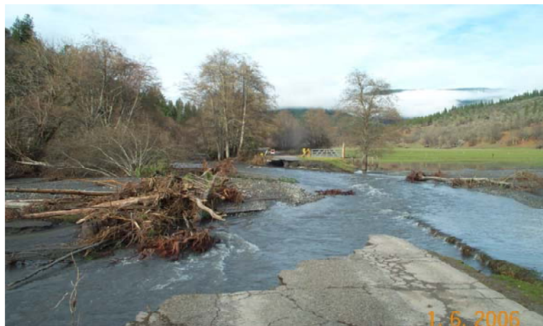
Figure 17: Damage to Bar Road caused by flooding in Horse Creek, January 2006.
