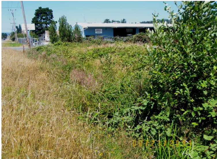
Figure 12: This drainage ditch that empties into Widow White Creek was equipped with check dams to catch sediment in conjunction with the pedestrian bridge project. Maintaining full vegetative cover in the ditch also reduces sediment delivery.
