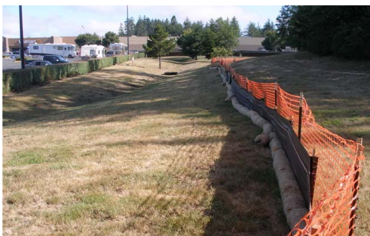
Figure 7: The swale on the left in the photograph conveys runoff from the development to three outfalls to an adjacent creek. In the top center of the photograph the entrance to an in-line treatment device is visible.
