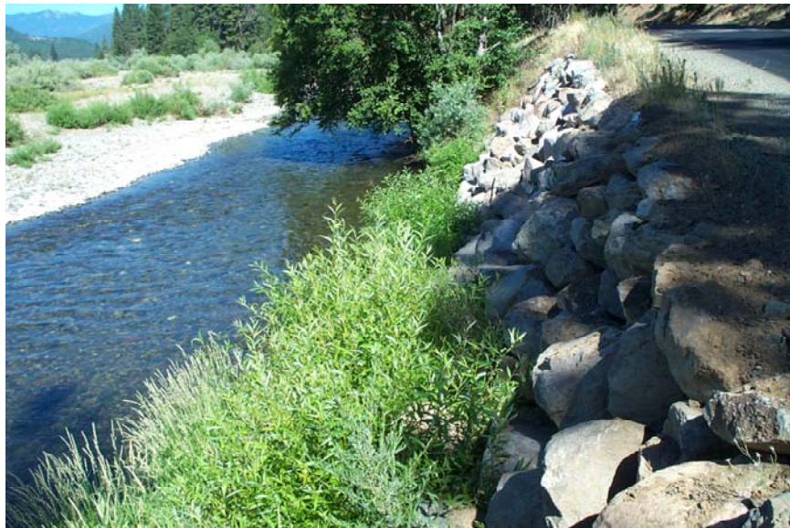
Figure 14: Bank stabilization on the Scott River Road utilizing a bioengineering approach. The site has remained stable for the past four years.
