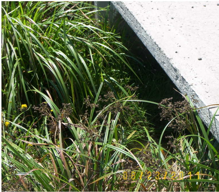
Figure 28: The entrance to the Crannell Road box culvert. Although the streambed was disturbed during removal of the old culvert and installation of the new one, it had completely revegetated naturally.
