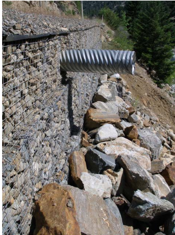
Figure 15: Retaining wall along Scott River Road above Scott River. Note rock slope protection applied at base of wall that also serves to dissipate energy from the culvert outfall.
