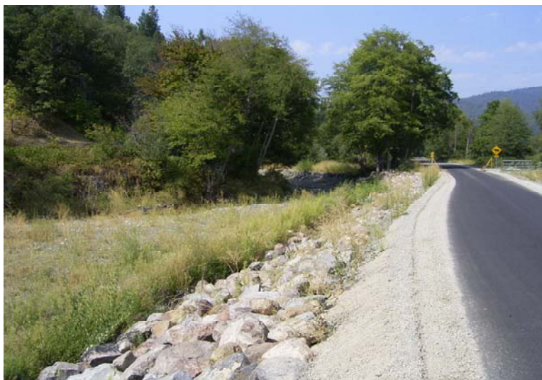
Figure 19: Rock slope protection and willow revegetation along Bar Road, one year after installation.
