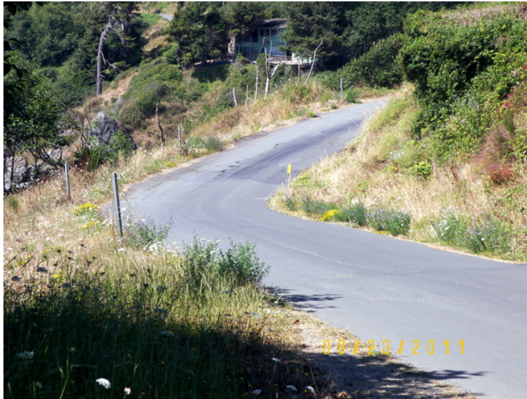
Figure 20: Section of Scenic Drive where failing road surface was repaired.
