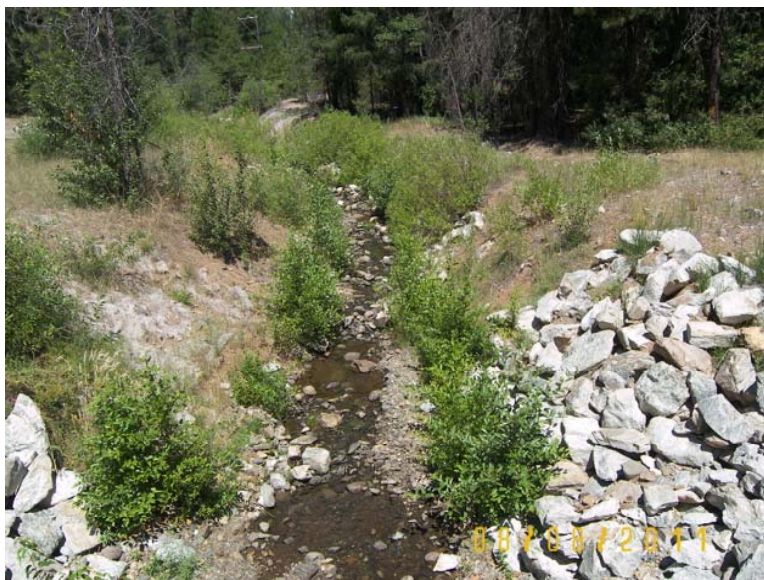
Figure 22: The channel upstream from the Little Brown's Creek bridge was engineered to promote fish passage and provide habitat structures. Banks were stabilized with rock and riparian plantings.
