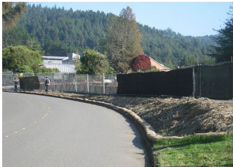
Figure 5: The corrected measures included addition of a coir roll along the disturbed site (above) and on the edge of the road across from the site (not shown).
