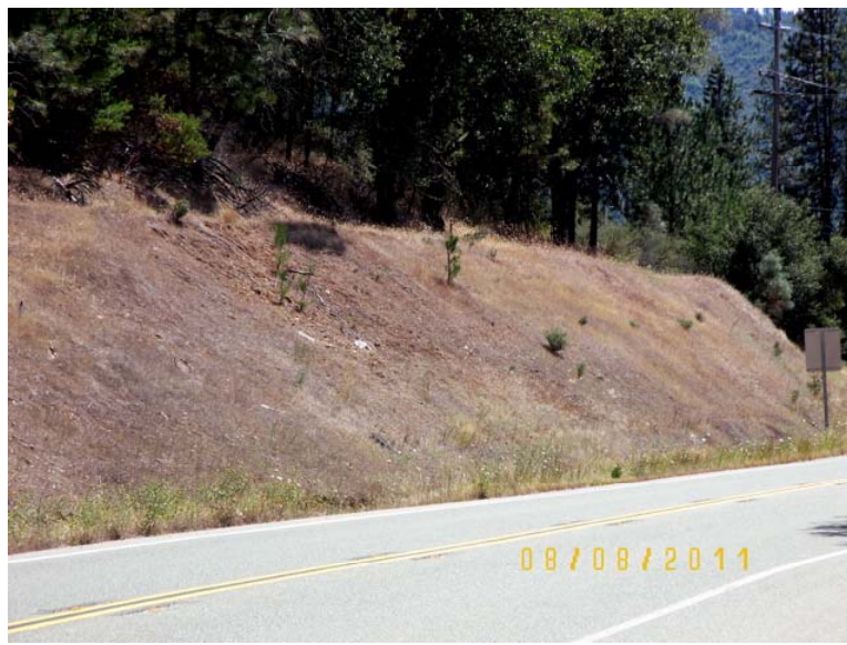
Figure 24: Cut slopes along the Rush Creek Road widening project were not fully revegetated after construction and were eroding, delivering sediment to the roadside ditch.
