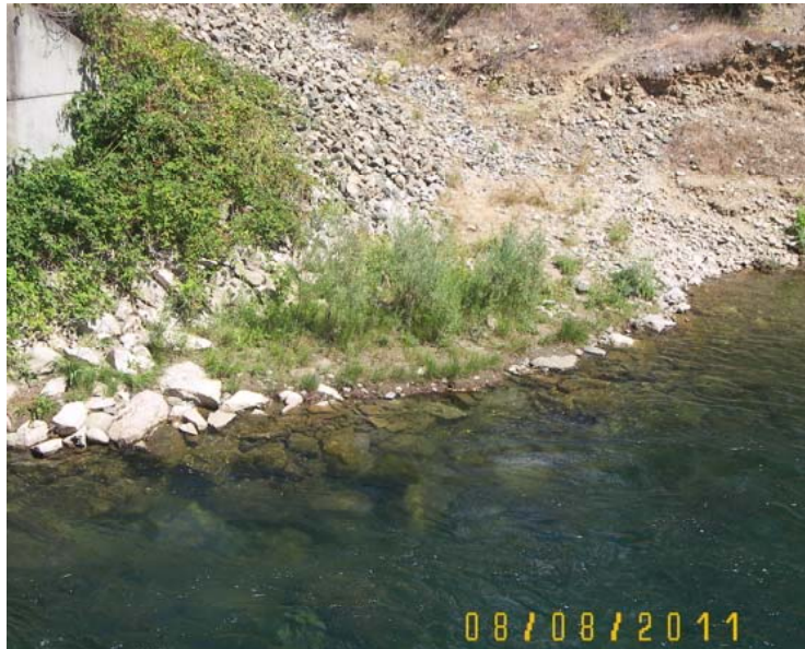
Figure 11: Rock slope protection placed at downstream end of Bucktail Bridge. The access ramp in the center of picture was rocked and blocked off to prevent vehicle access.
