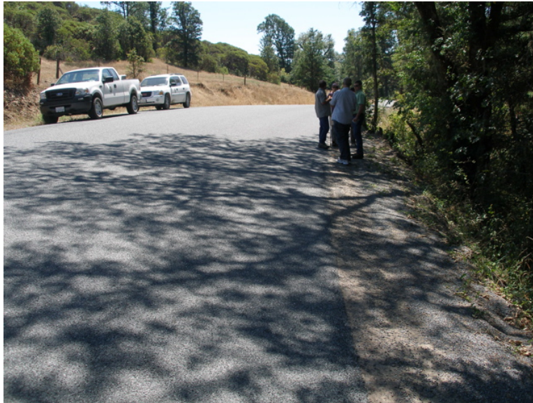
Figure 23: Chip sealing and outsloping on the Tomki Road, Mendocino County.
