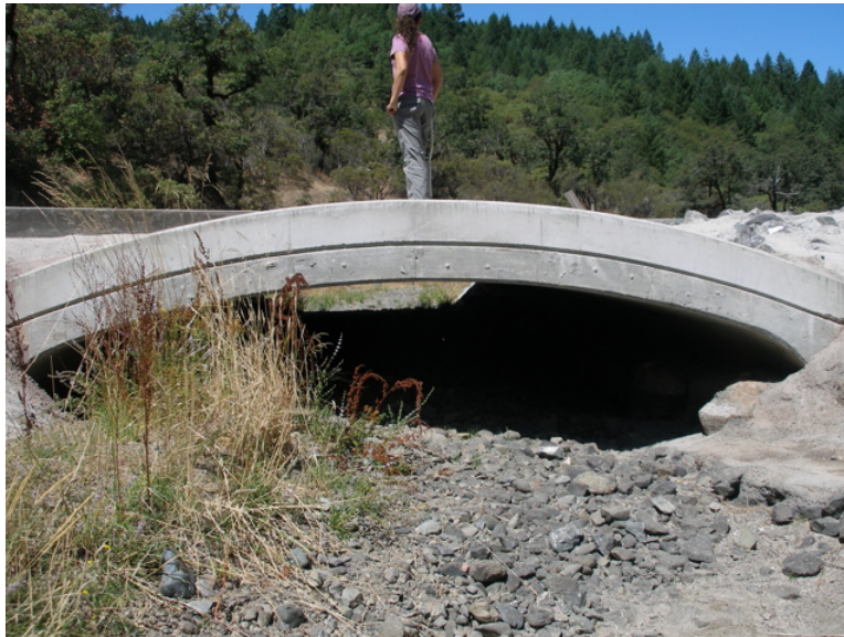
Figure 26: Tomki Road vented ford. The bottomless arch is surrounded by concrete to prevent undermining and erosion.
