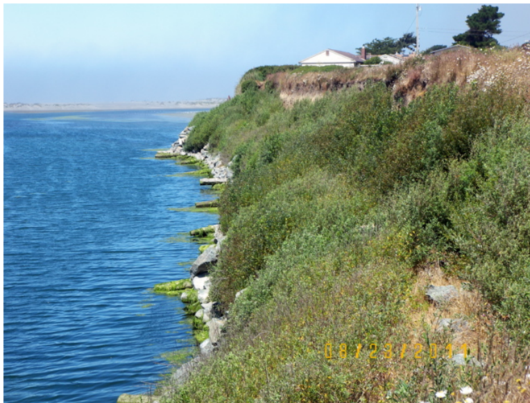
Figure 16: Bioengineered bank stabilization on the Mad River.
