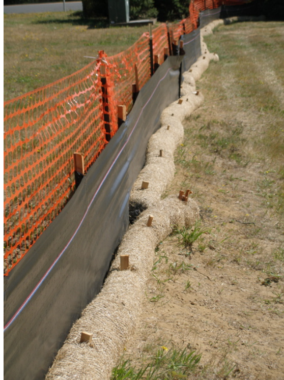
Figure 3: At this commercial site in Del Norte County staked straw rolls and a silt fence were in place along the entire boundary between an adjacent creek and the development (August 2011). We also observed similar measures in place at stockpiled soil.
