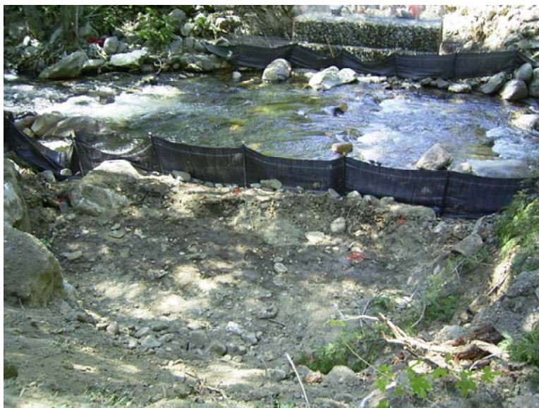
Figure 13: Silt fence installed at a bridge replacement site to prevent sedimentation in the stream.
