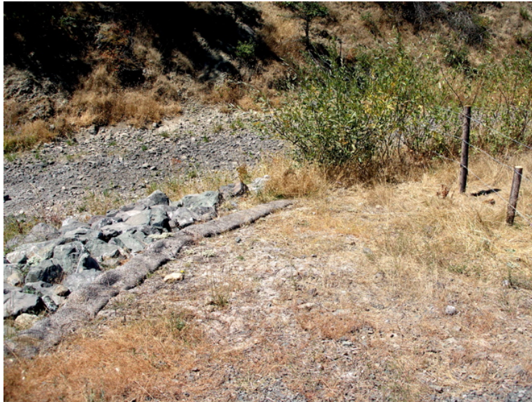
Figure 27: Streambank stabilization and riparian planting at the Tomki Road vented ford.
