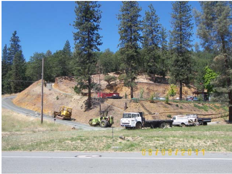
Figure 6: Unregulated grading near Weaverville, Trinity County. This site has been of considerable interest to the Regional Water Board.
