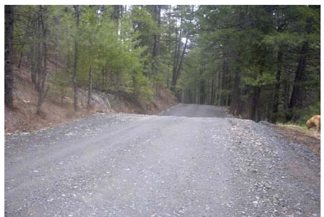
Photo G (Lower left). China Gulch Road showing both ditch and cutbank erosion. Photo H (Lower right). China Gulch Road after ditch removal showing outslope and exaggerated rolling dip. The exaggerated dips were used due to the cutbank slides on and low vehicle use of the road.
