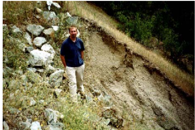
Photo A (Upper left). Trinity Alps Road fill failure in May 2003. The combination of decomposed granitic soils and saturated fill resulted in the fill failure at this Class III stream crossing. Photo B (Upper right). Trinity Dam Boulevard showing fill erosion in May 2003 from diverted road surface runoff.
