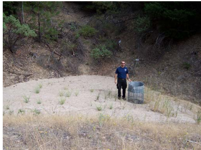
Photo C (Lower left). Trinity Dam Boulevard showing cutbank sediment delivery to a ditch. Photo D (Lower right) showing sediment delivery from a ditch to a sediment basin and a culvert inlet. Periodic removal of sediment from basins can reduce delivery to streams.
