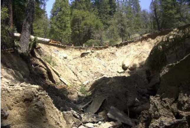
Photo A (Upper left). Trinity Alps Road fill failure in May 2003. The combination of decomposed granitic soils and saturated fill resulted in the fill failure at this Class III stream crossing. Photo B (Upper right). Trinity Dam Boulevard showing fill erosion in May 2003 from diverted road surface runoff.
