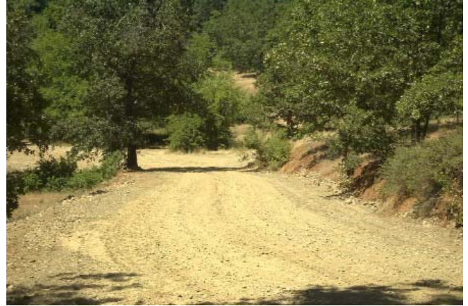
Photo E (Upper left). Dutch Creek Road showing diverted ditch flow down road. Photo F (Upper right). Same location after the road was outsloped with rolling dips and rock surfacing.
