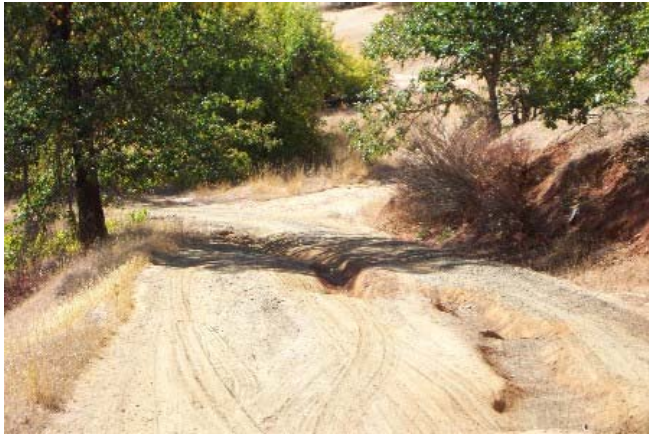
Photo E (Upper left). Dutch Creek Road showing diverted ditch flow down road. Photo F (Upper right). Same location after the road was outsloped with rolling dips and rock surfacing.
