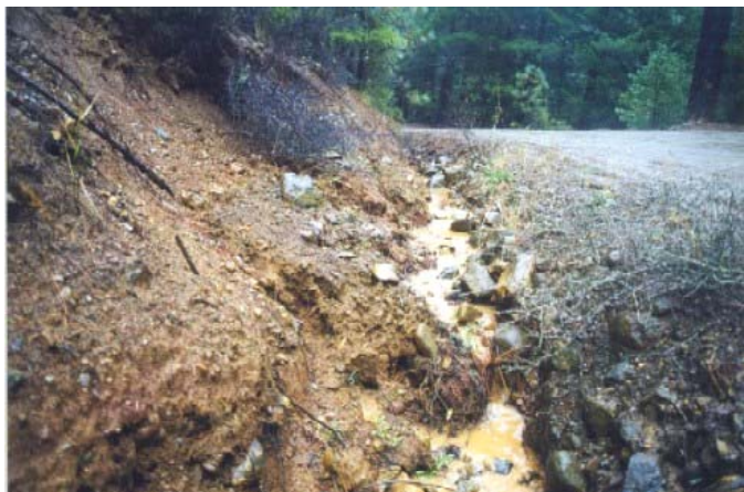
Photo G (Lower left). China Gulch Road showing both ditch and cutbank erosion. Photo H (Lower right). China Gulch Road after ditch removal showing outslope and exaggerated rolling dip. The exaggerated dips were used due to the cutbank slides on and low vehicle use of the road.
