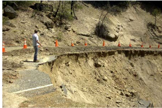
Photo 1 and 2. Trinity Alps Resort Road fill failure in decomposed granite soils. May 2003
