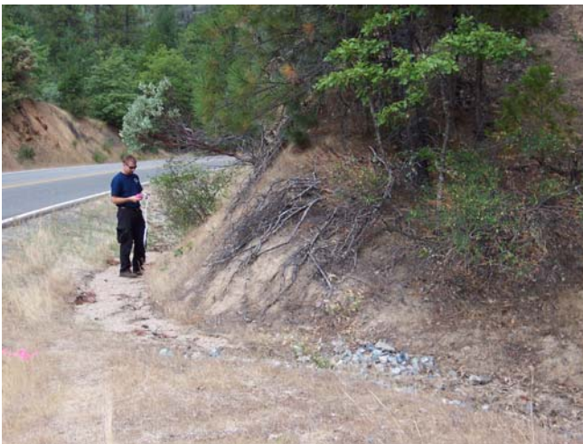
Photo C (Lower left). Trinity Dam Boulevard showing cutbank sediment delivery to a ditch. Photo D (Lower right) showing sediment delivery from a ditch to a sediment basin and a culvert inlet. Periodic removal of sediment from basins can reduce delivery to streams.
