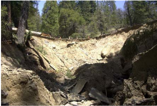
Photo 1 and 2. Trinity Alps Resort Road fill failure in decomposed granite soils. May 2003
