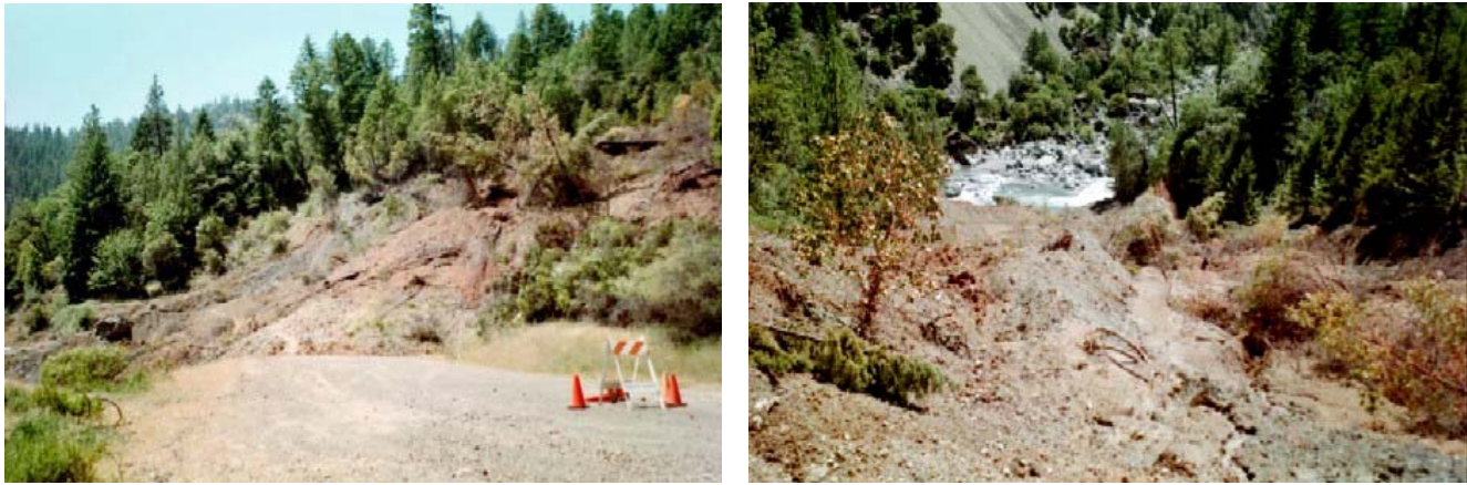
Big Slide on Lower South Fork Road in Hyampom above the South Fork of the Trinity River. Road crews have been removing material as part of their efforts to re-open the road. The failure volume of the most recent event was estimated at ~ 231,000 yd 3 – much higher than that originally projected (1,952 yd 3 ). Of that ~ 45,000 yd 3 is thought to have delivered to the South Fork Trinity River. (Figures obtained from USDA Forest Service “Big Slide near Hyampom Mass Failure Report, January 24, 2003.”)
