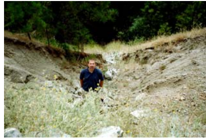
Trinity Drinking Water Source Sediment Reduction Project Roads- Left: Browns Mountain Road with plugged and diverted culvert Right: Past outboard fill failure on Trinity Dam Boulevard
