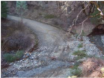
Trinity Drinking Water Source Sediment Reduction Project Roads- Left: Browns Mountain Road with plugged and diverted culvert Right: Past outboard fill failure on Trinity Dam Boulevard
