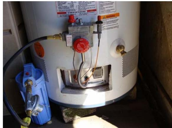
**Above:** Methane & CO<sub>2</sub> gas captured & burned to heat water & dry clothes on a dairy farm, Del Norte County
