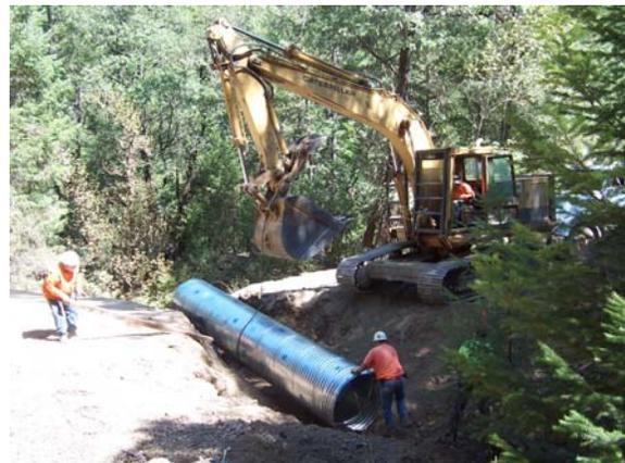
**Upper Left:** Installing a new culvert with armored outboard fill on Indian Creek Road (2008)
