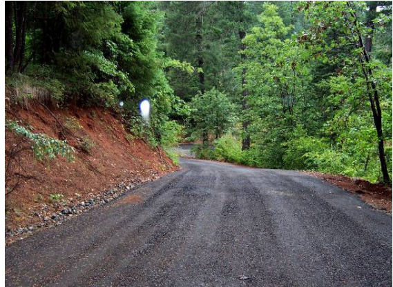
China Gulch Road Post-Project (Lancaster) 2012. Photo taken during winter storm
