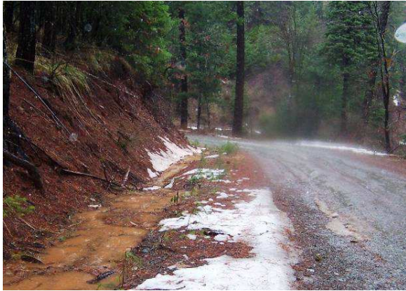
China Gulch Road Pre-Project (Lancaster) 2004. Photo taken during winter storm
