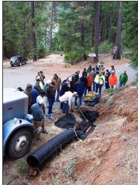
2012 Roads Workshop sediment control sock/bag demonstration (Colbeck)
