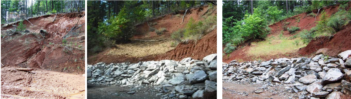
Photo documentation on Dutch Creek Road
