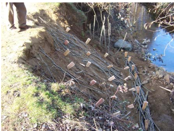
Figures 2 &3: Pilot bioengineering treatment on an eroding bank of Sidney Gulch in Trinity County shown as built in 2007 and one year later.
