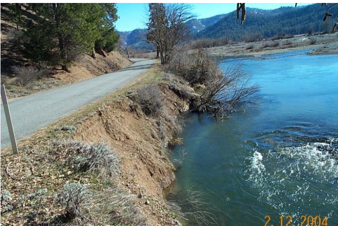
Figures 6 & 7: The pictures above illustrate a bioengineering project on the Scott River in Siskiyou County. Road Manual BMP 7.3 (Bioengineering Joint Planting) was used to stabilize an eroding bank.
