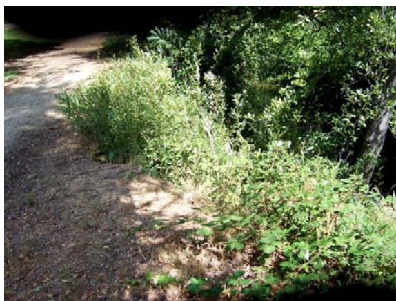
Figures 2 &3: Pilot bioengineering treatment on an eroding bank of Sidney Gulch in Trinity County shown as built in 2007 and one year later.
