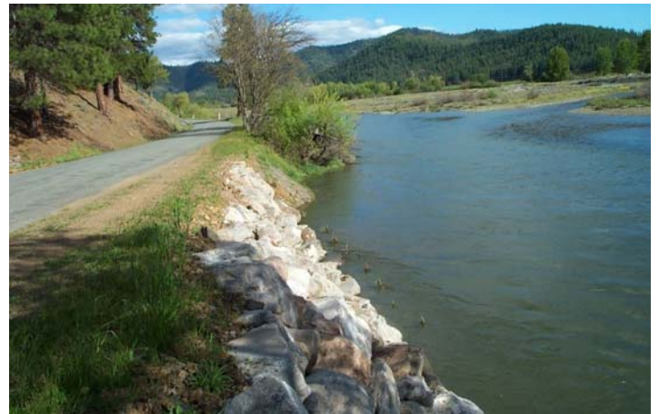
Figures 6 & 7: The pictures above illustrate a bioengineering project on the Scott River in Siskiyou County. Road Manual BMP 7.3 (Bioengineering Joint Planting) was used to stabilize an eroding bank.
