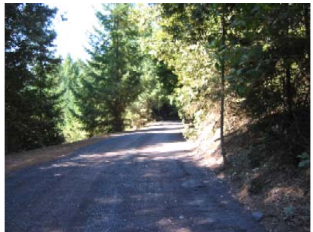
Figure Set 13: Mendocino County project site with in-board ditch and native road surface (above left). Above right, same location after out-sloping, rocking with PermaZyme treatment.
