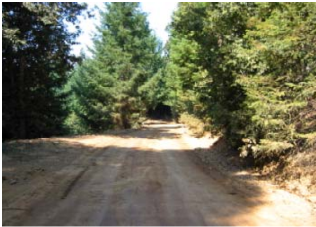
Figure Set 13: Mendocino County project site with in-board ditch and native road surface (above left). Above right, same location after out-sloping, rocking with PermaZyme treatment.
