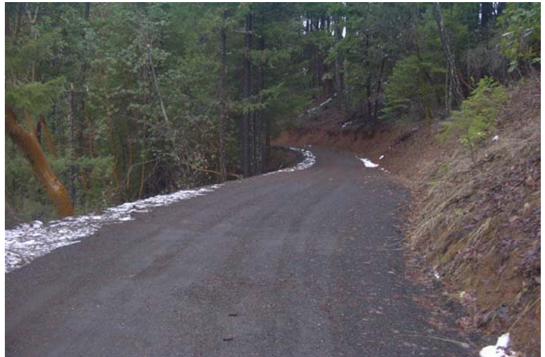
Figure 9: Recycled AC grindings on Dutch Creek Rd (Trinity County)
