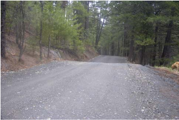
Figure Set 10: Left- LITH road with rolling dip and outslope drainage. Right- Same road prior to modification with in board ditch and in-slope configuration.
