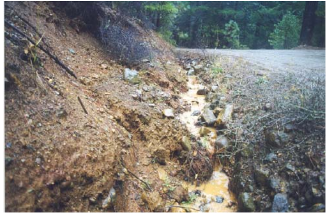
Figure Set 10: Left- LITH road with rolling dip and outslope drainage. Right- Same road prior to modification with in board ditch and in-slope configuration.
