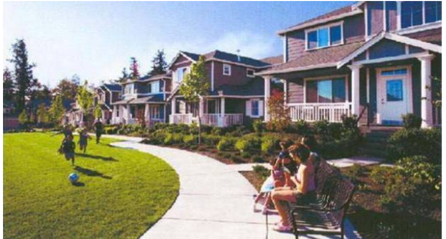
Figure 1. Compost amendment of disturbed soils reduces long-term maintenance and irrigation, reducing or eliminating the need for pesticides and herbicides.
