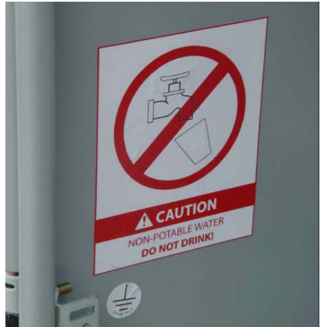
Figure 7 Stickers remind users that untreated cistern water is not safe to drink without treating.
