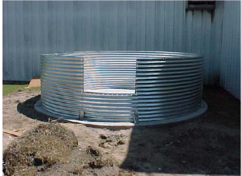
Figure 3 Metal cistern being constructed.
