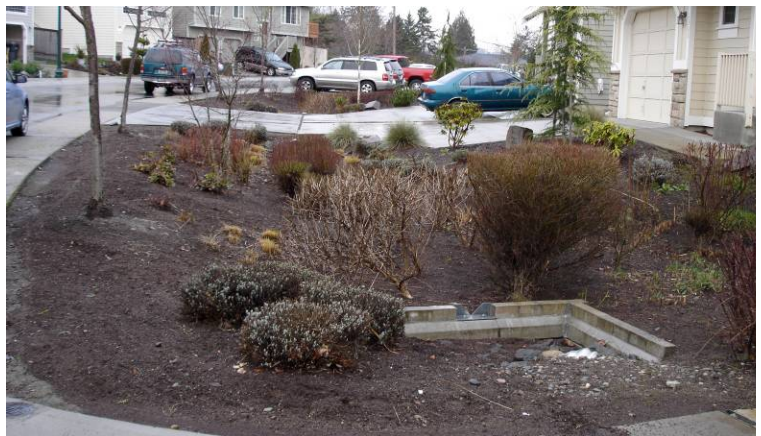
Figure 7 Rain gardens are great alternative to manage runoff when it can't be prevented.
