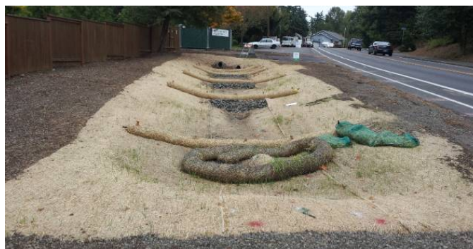
Figure 11 Even a single practice like this rain garden will need additional BMPs implemented (erosion control) to be really effective long-term.
