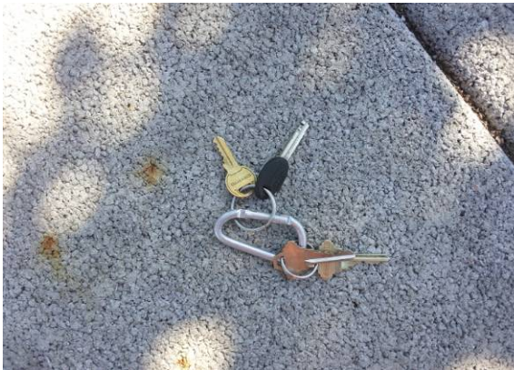
Figure 4 Pervious concrete infiltrates rainfall at the source.
