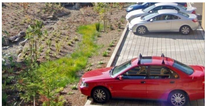
Figure 10 A daylight stream, a rain garden, porous pavement, and native plants all work together to protect water resources on and off site.
