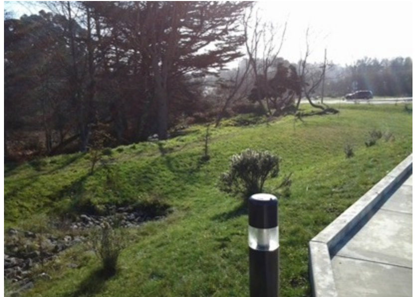
Figure 1. A vegetated swale can be an aesthetically pleasing way to convey water around a site and protect downstream waterways.
