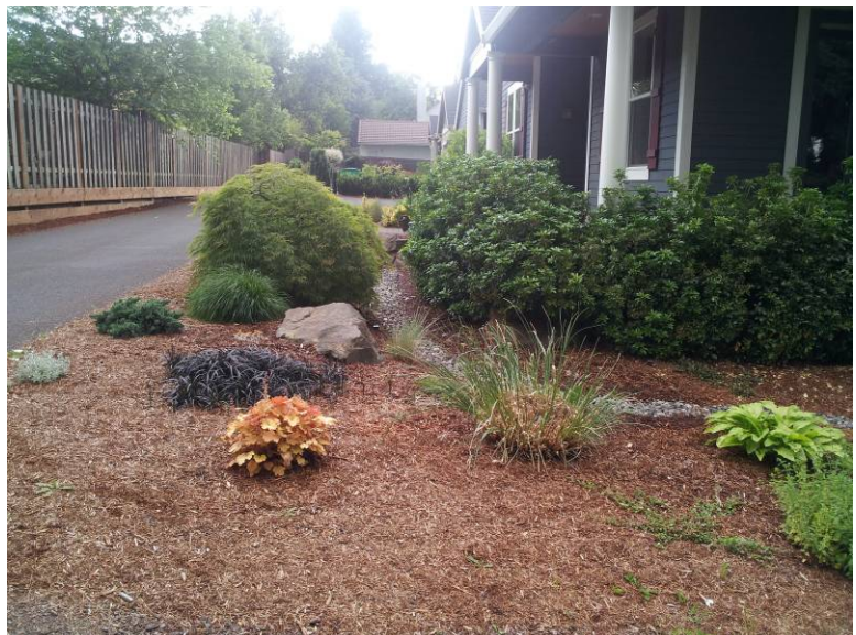
Figure 10. Rock swale conveys water from a downspout
