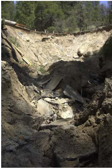
Photos 1 and 2. Trinity Alps Road fill failure in May 2003. The combination of decomposed granitic soils, improper road drainage and saturated fill resulted in the fill failure at this Class III stream crossing.
