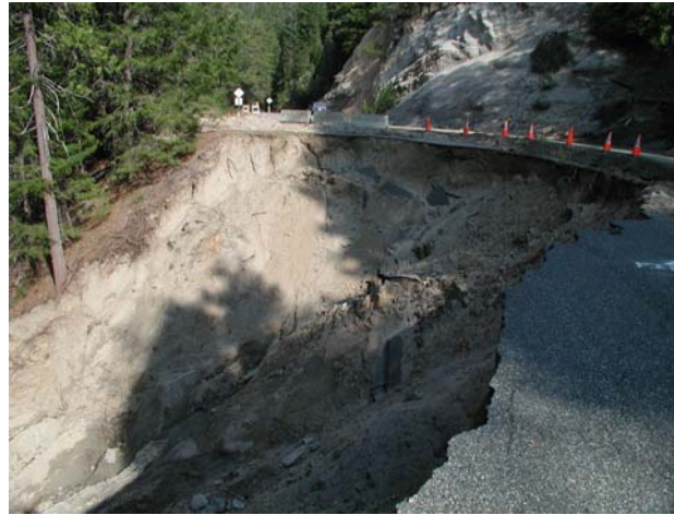
Photos 1 and 2. Trinity Alps Road fill failure in May 2003. The combination of decomposed granitic soils, improper road drainage and saturated fill resulted in the fill failure at this Class III stream crossing.
