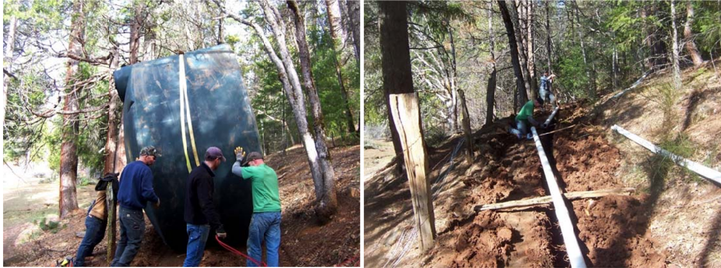
Figure 20 & 21- The 5,000 gallon water tanks were rolled up a narrow trail above the pasture (left) and the 4" return flow line was placed in the center of the trail (right).
