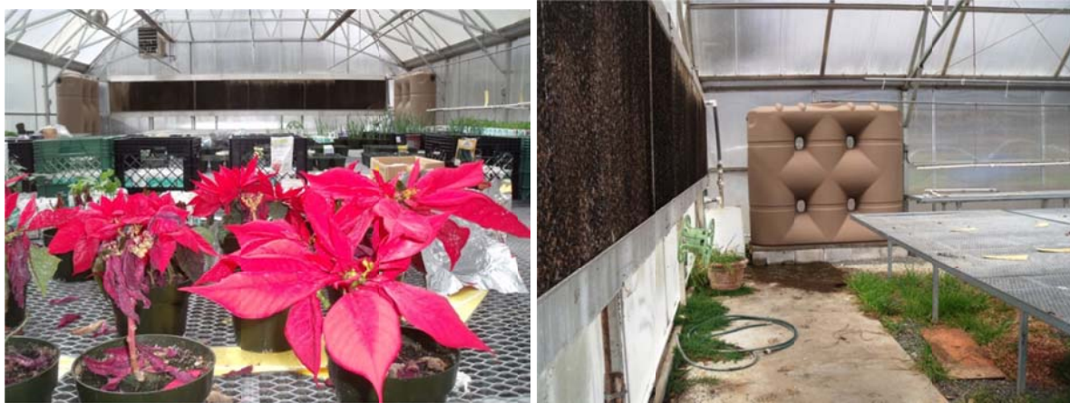
Figures 10, 11 & 12: Trinity High School's greenhouse program's largest tank is located outside of the greenhouse (above left and right). The exterior system includes a rainwater diverter and diffuser, overflow system and discharge pipe and one way valves (above middle). The interior tanks ( Figure 13 & 14 below) warm water and provide thermal mass to the greenhouse. The greenhouse roof yields ~750 gallons of water per inch of rainfall.
