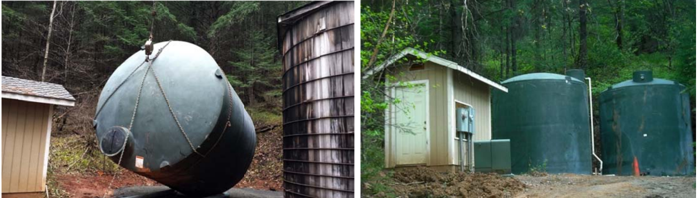
Figure 17 & 18- The 13.6' tall tanks were placed with a lift. The first tank was placed with redwood tank still providing community water (left). Once testing of the new tank and water was complete the redwood tank was removed and the second tank set (right).
