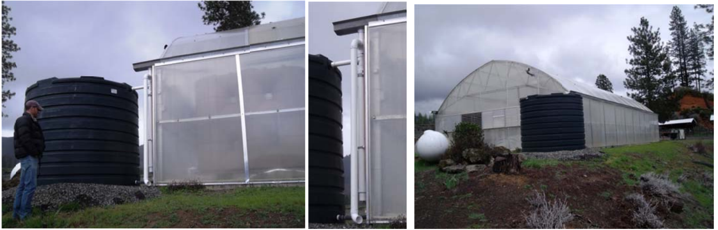
Figures 10, 11 & 12: Trinity High School's greenhouse program's largest tank is located outside of the greenhouse (above left and right). The exterior system includes a rainwater diverter and diffuser, overflow system and discharge pipe and one way valves (above middle). The interior tanks ( Figure 13 & 14 below) warm water and provide thermal mass to the greenhouse. The greenhouse roof yields ~750 gallons of water per inch of rainfall.
