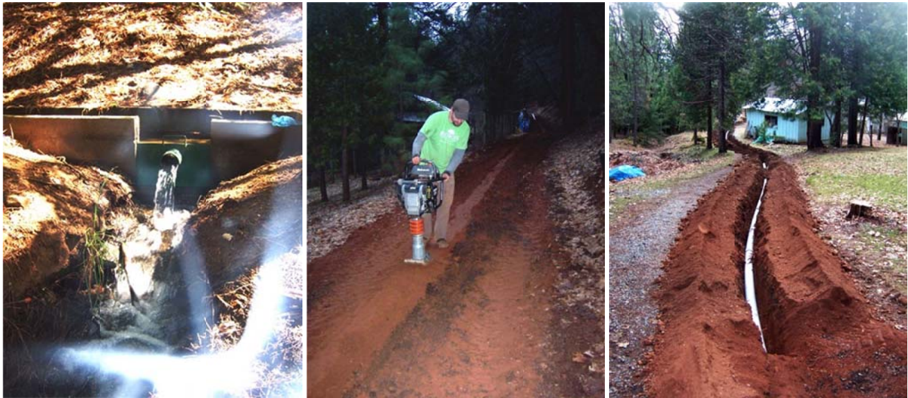
Figure 22 – 24- The Ditch flow in the summer of 2013 prior to project initiation (left), the return flow line trench was installed in the trail (middle) and main driveway (left). The trench was compacted and road rock replaced following installation of the water line.
