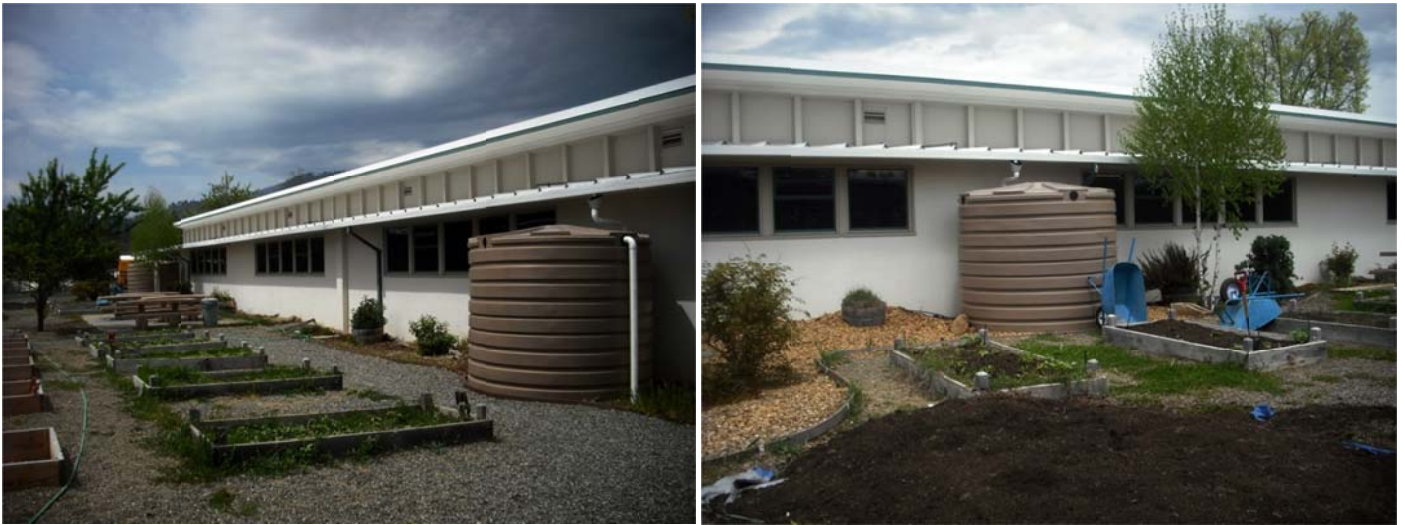
Figures 15 & 16- Weaverville Elementary School Childrens Garden Rooftop rainwater tanks are integrated into the garden space. All garden water will come from rainwater collection beginning in 2014.
