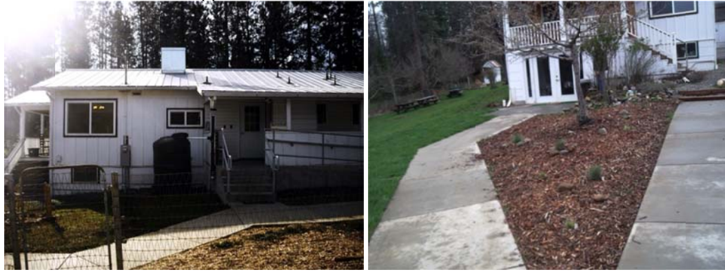
Figure 24 & 25: A 500 gallon water tank collects rooftop rainwater from the Young Family Ranch roof. Water collected in this tank is used on the lawn and drought landscaping (Above right) installed as part of the March 8 th , 2014 water conservation workshop held at the Ranch.
