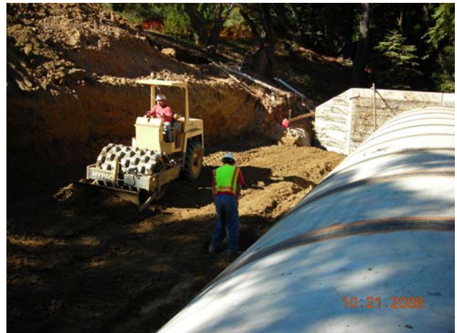
Bringing up structural backfill on Marsh Creek.
