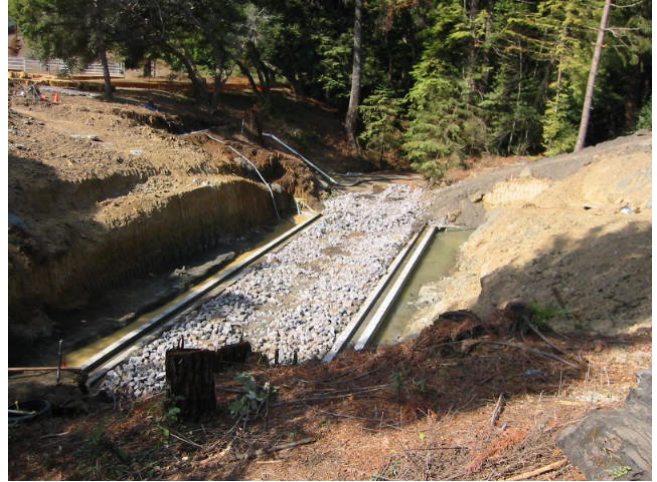
Finished strip footing on Marsh Creek.
