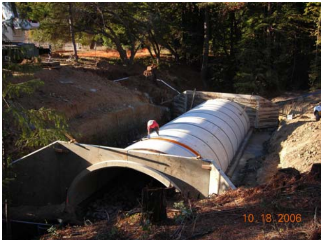
Structure water proofing on Marsh Creek.
