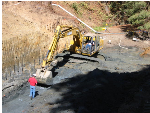
Digging the footings on Marsh Creek.
