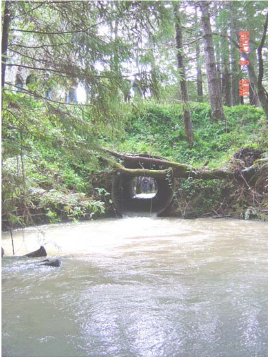
Marsh Creek outlet before new structure
