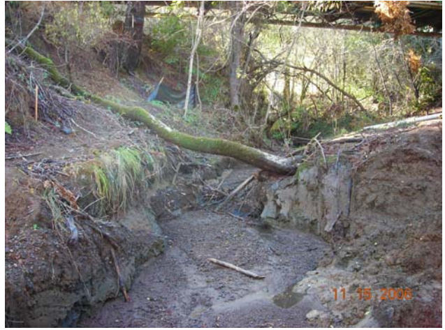
Looking upstream from the Marsh Creek inlet. Channel is responding by head cutting upstream and banks collapsing in resulting in a wider channel to accommodate the new structure (no more restrictions).
