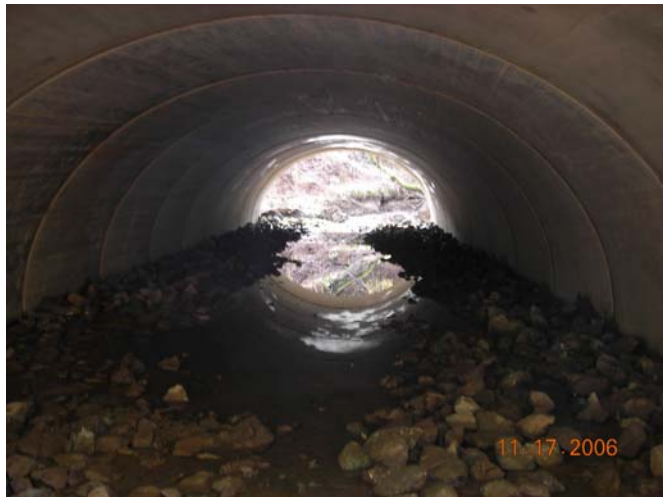
Marsh Creek new structure
