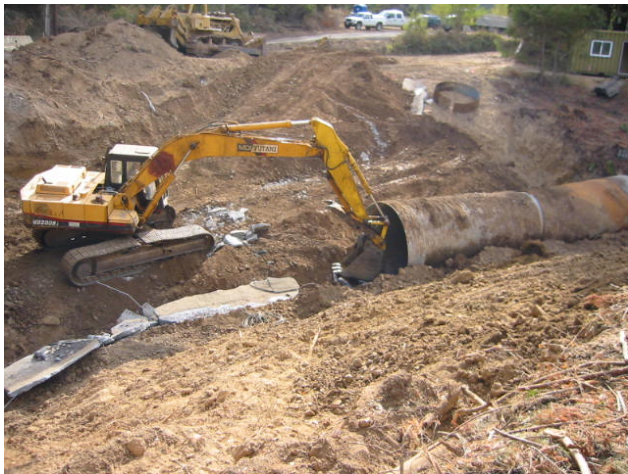
Removing the old culvert on Marsh Creek.
