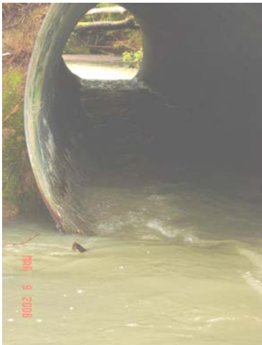
Marsh Creek before new structure
