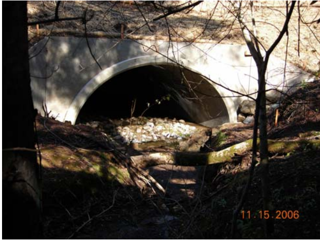
Marsh Creek inlet after completion.
