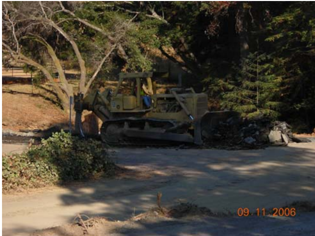
Tearing out the pavement on Marsh Creek.
