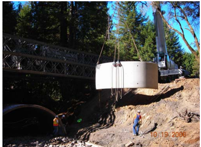
Lowering arch elements in place on the Albion.
