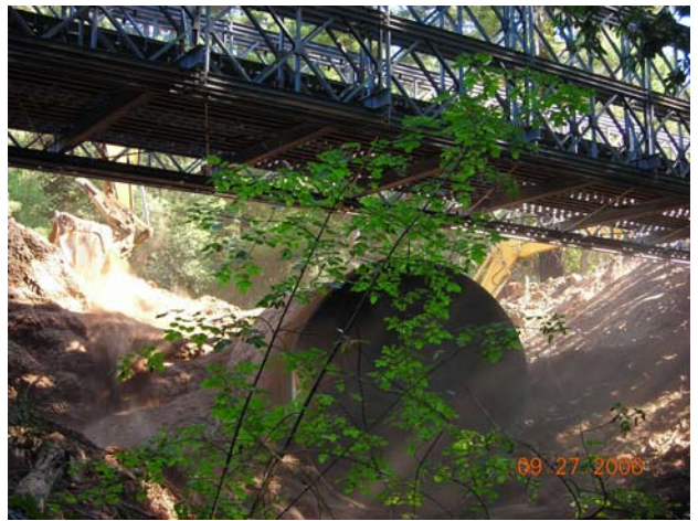
Excavation underway on the Albion.
