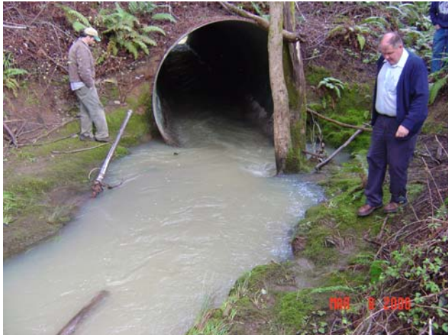
Marsh Creek Inlet before new structure
