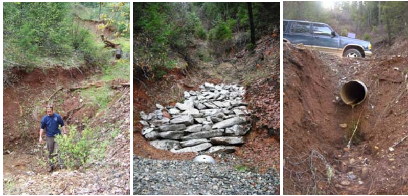
Buried wood in the outboard fill as well as accumulated surface wood (below left). Excavating to remove old culvert, woody debris and fill (middle). Installed 60' x 24" culvert set near channel gradient (~14' below road grade) with critical dip and RSP installed (right).
