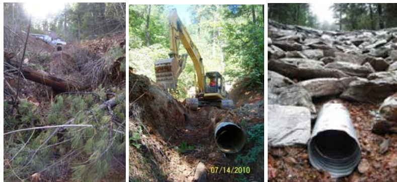
Buried wood in the outboard fill as well as accumulated surface wood (below left). Excavating to remove old culvert, woody debris and fill (middle). Installed 60' x 24" culvert set near channel gradient (~14' below road grade) with critical dip and RSP installed (right).
