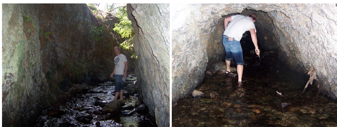
Figure 1 – Cut through 18 ft. of schist parent material (Left) Figure 2 – Tunnel under Quail Rd. (Right).
