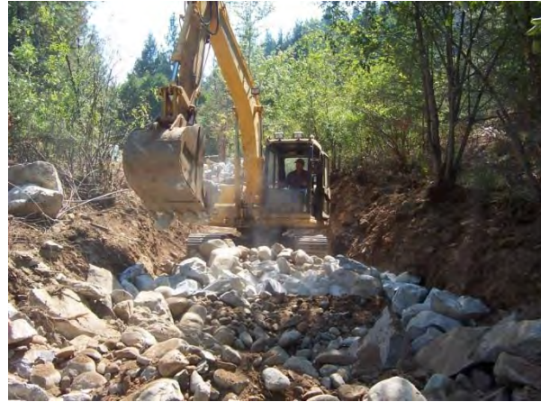
Figure 7-5: Installation of stream bed materials.
