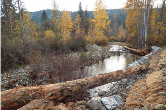
Figure 6-2: Engineered large wood installed in the lower reaches of East Weaver Creek in November 2014.
