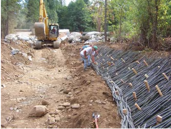
Figure 7-8: Willow mattresses before soil is added to them.
