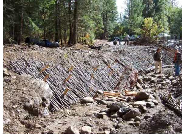
Figure 7-9: Willow walls and bed
