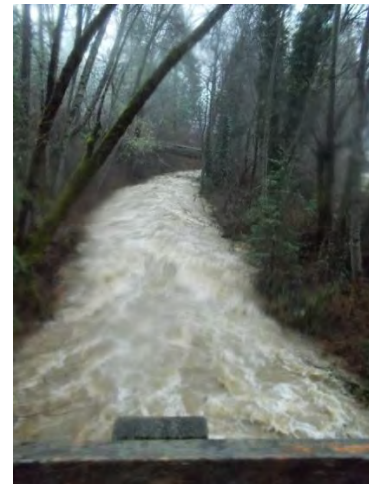
Figure 10-7: Storm flows from Butterfield Pedestrian Bridge in January 2016. The Bonar Bridge is visible.
