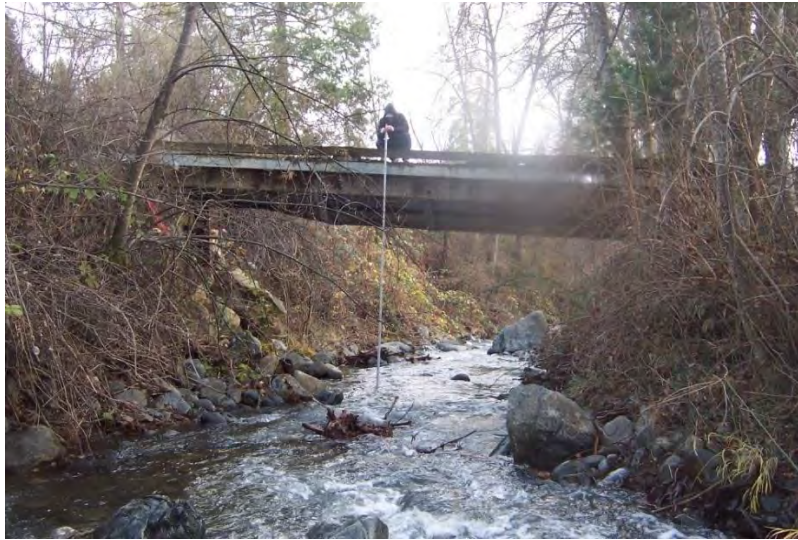
Figure 10-8: Bonar Private Road Bridge in December 2015.
