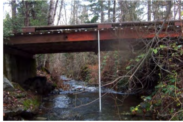
Figure 10-3: Hansen Mine Bridge spans the entire floodplain of East Weaver Creek
