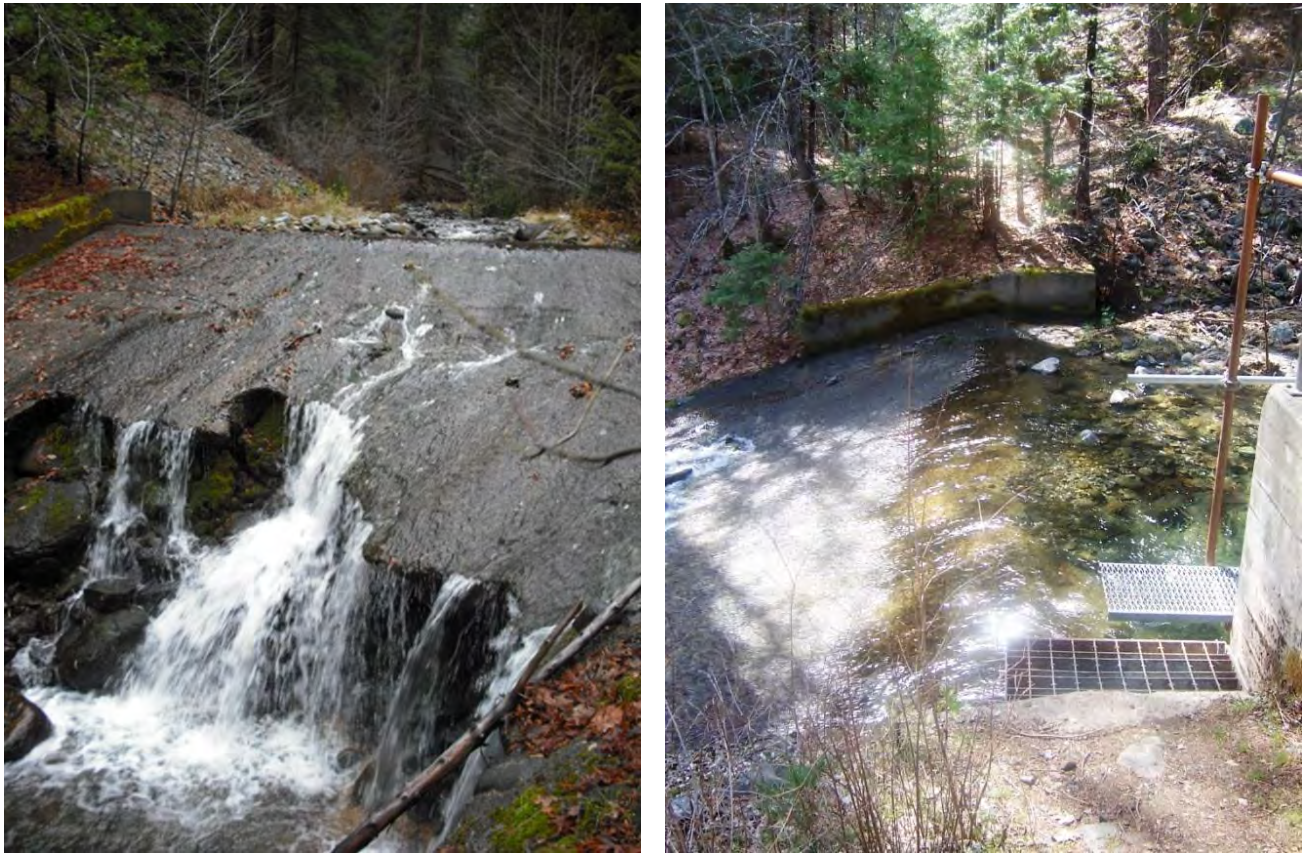
Figure 2-3. Dam showing concrete cap (left) and stilling basin to the EWF (right).
