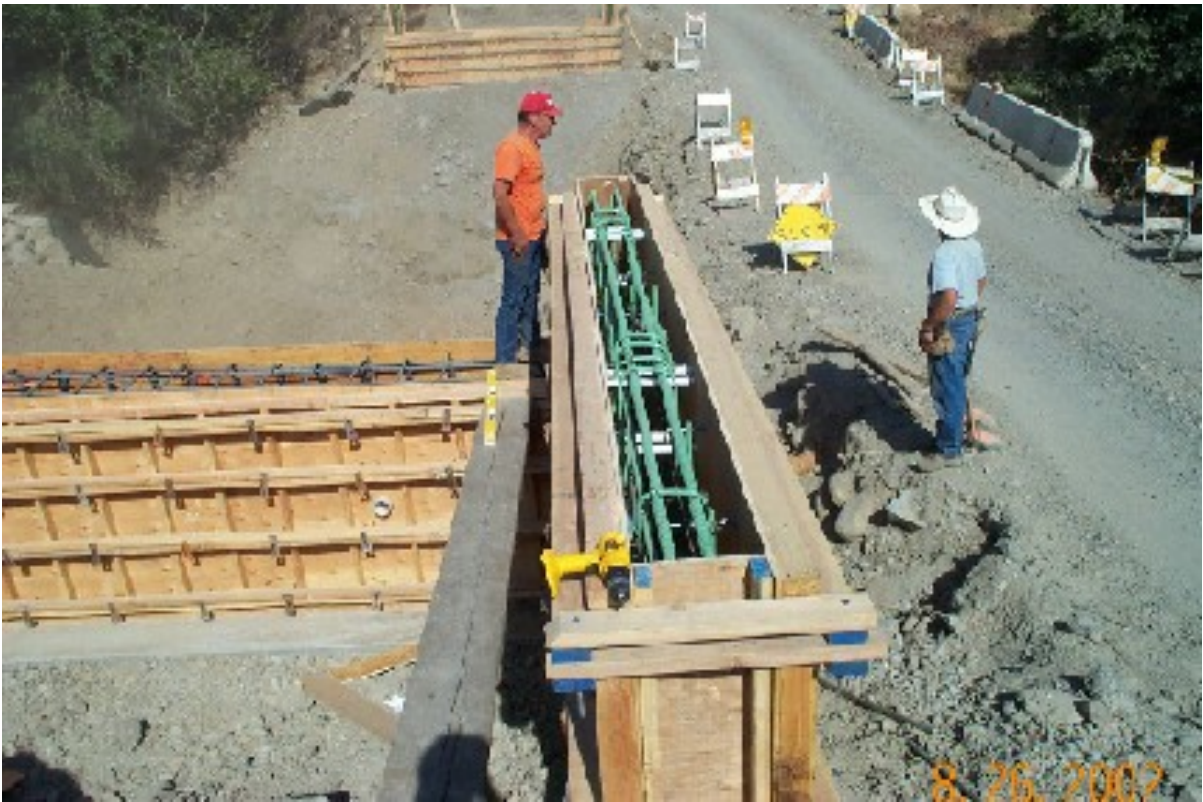
Epoxy coated rebar in tops of wing walls
