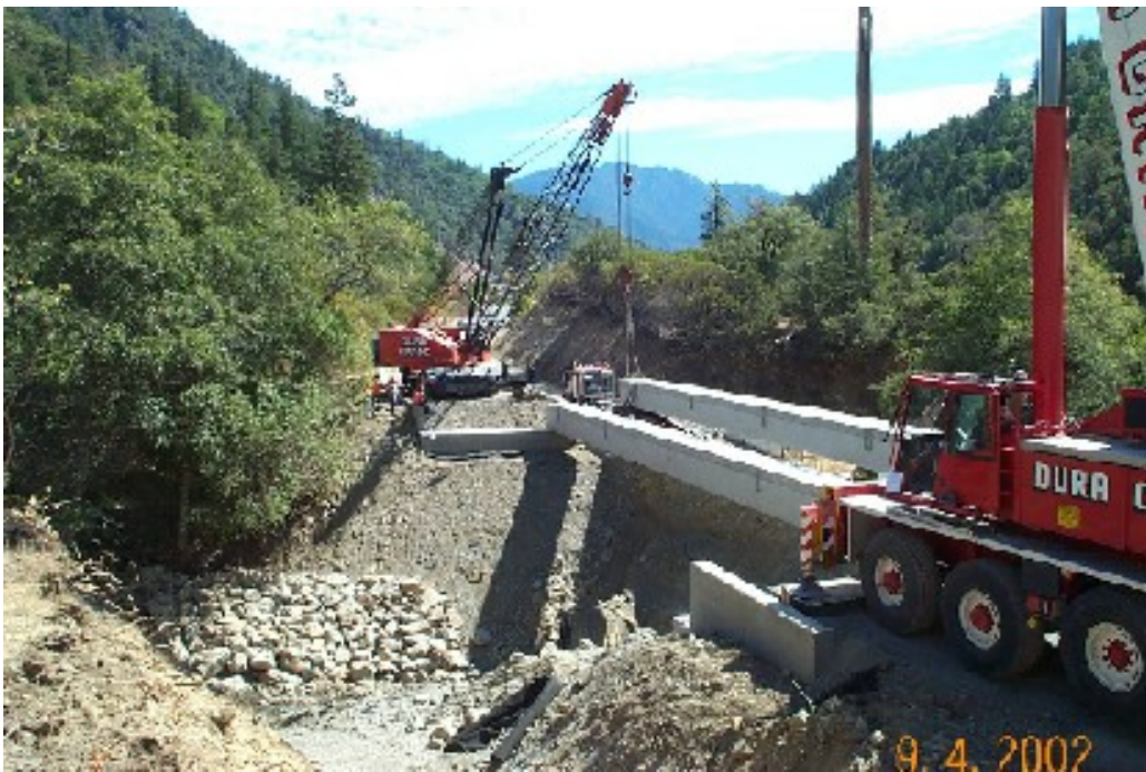
Setting box girders in place with two cranes
