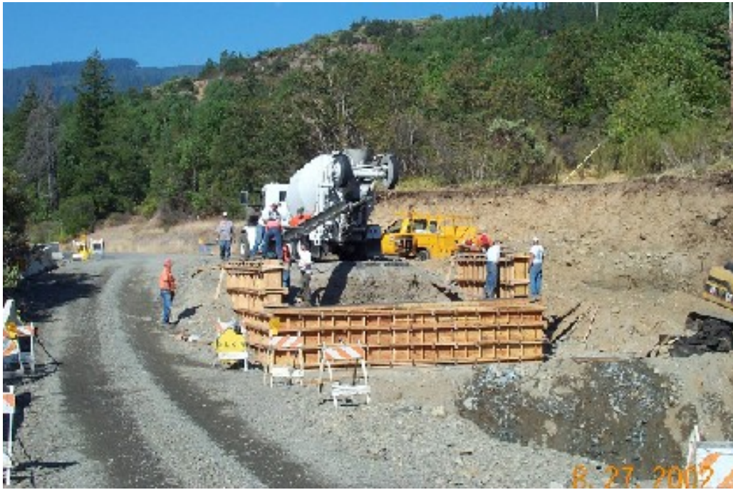
Dry batch method used for abutment pours
