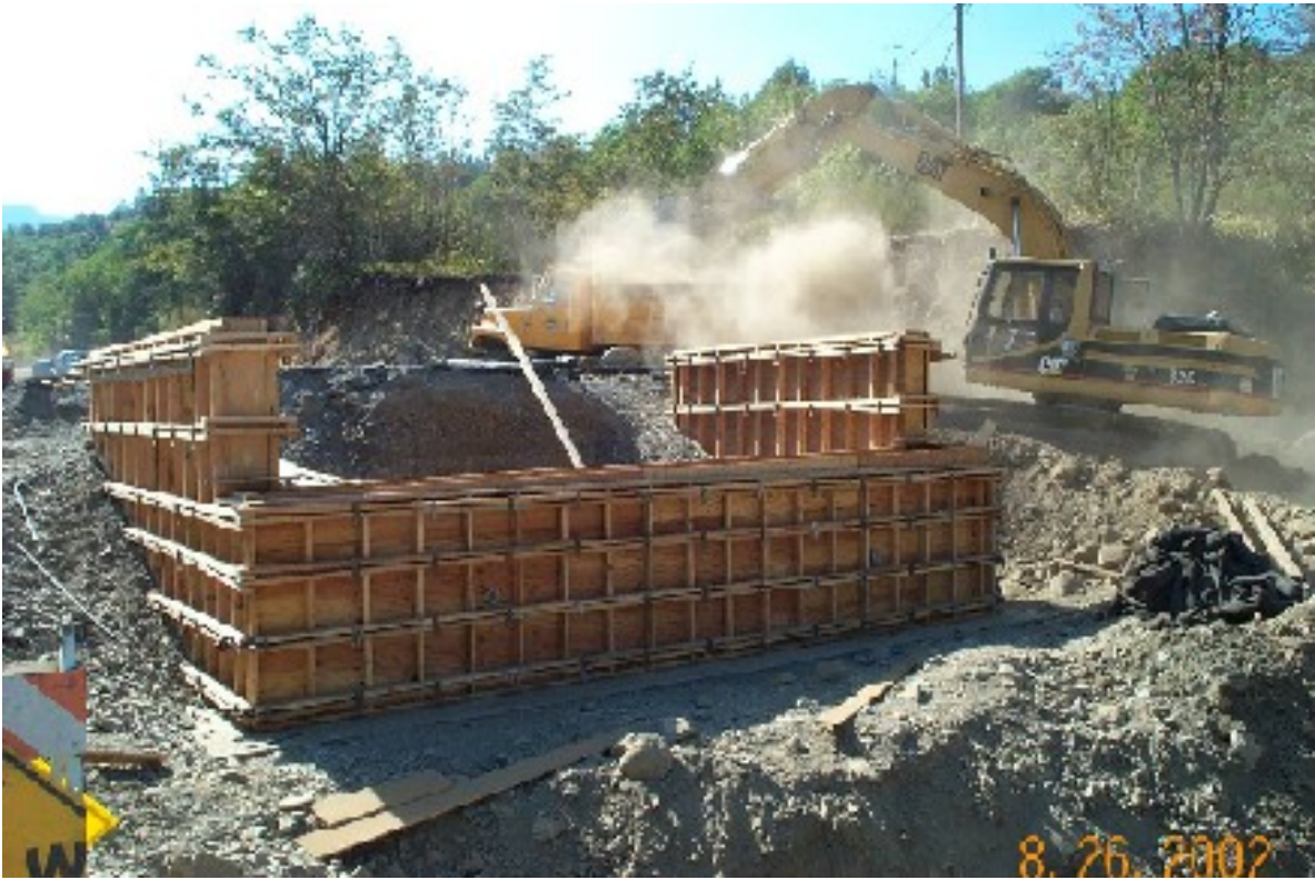
Forming abutments and wing walls on caps
