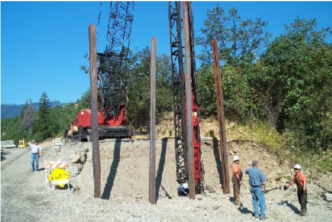
Driving eight 70 ton H-piles, front four battered at each abutment
