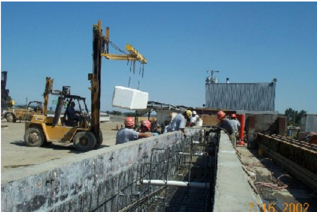
Forming box girders at casting plant
