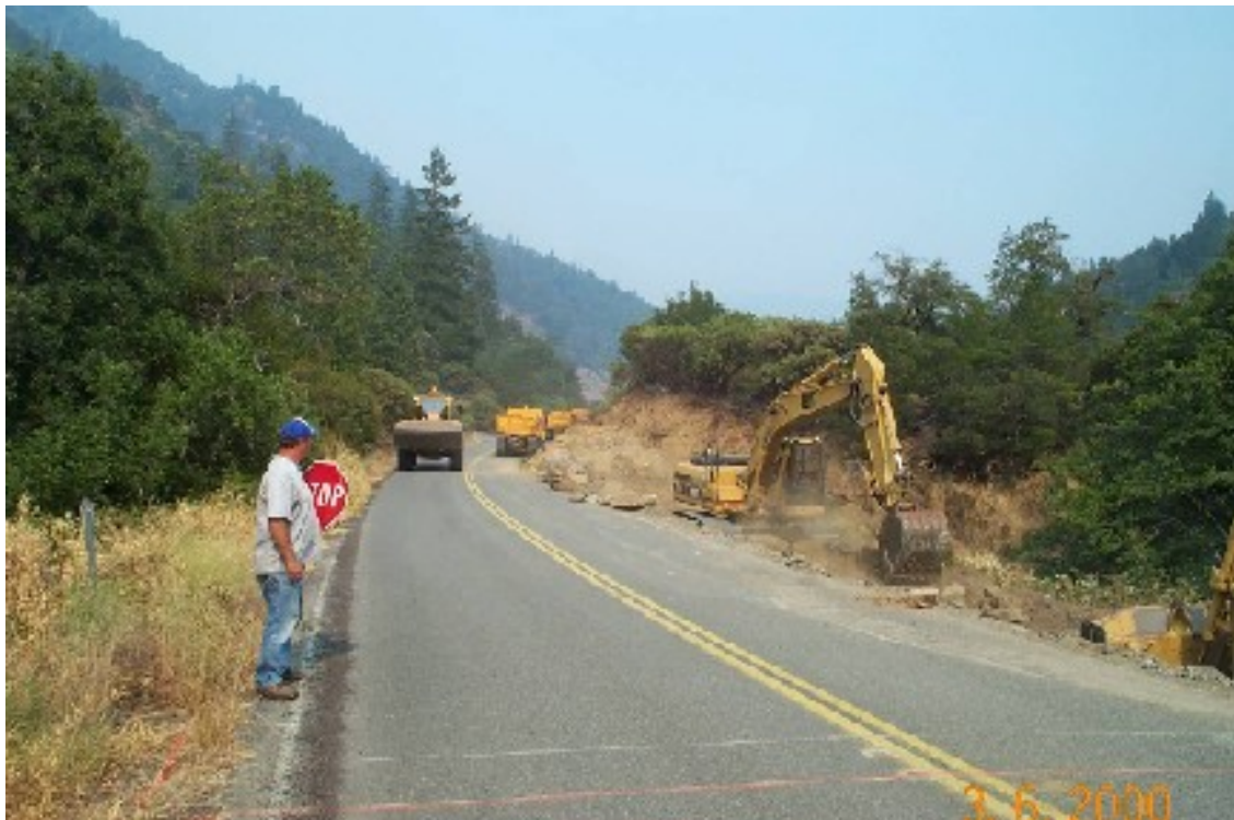
Construction begins by excavating for detour
