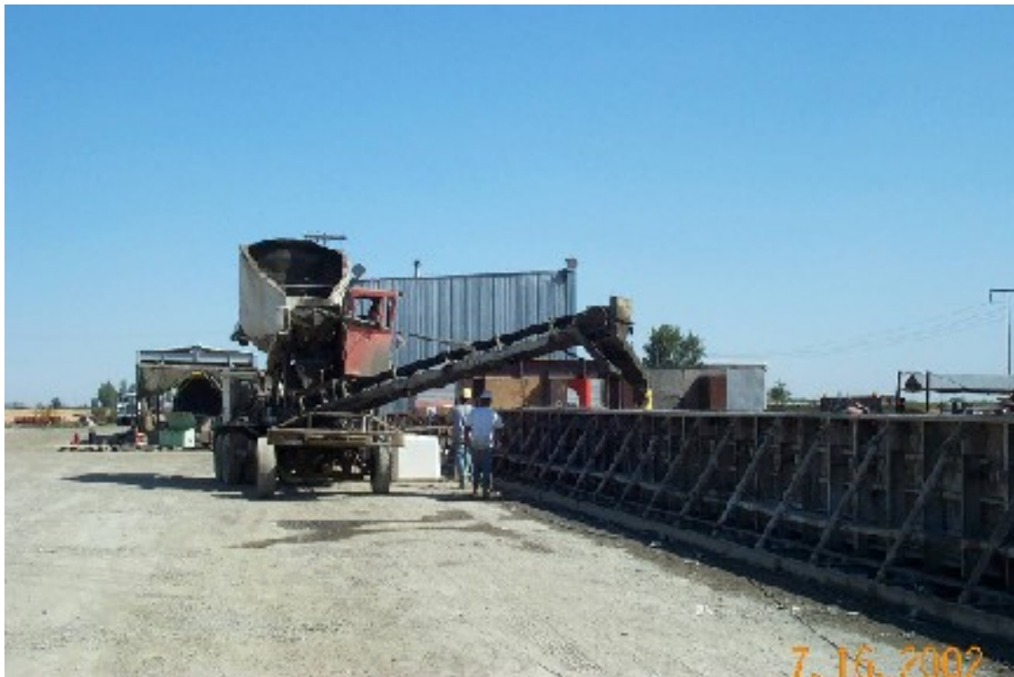
Placing concrete in box girder forms
