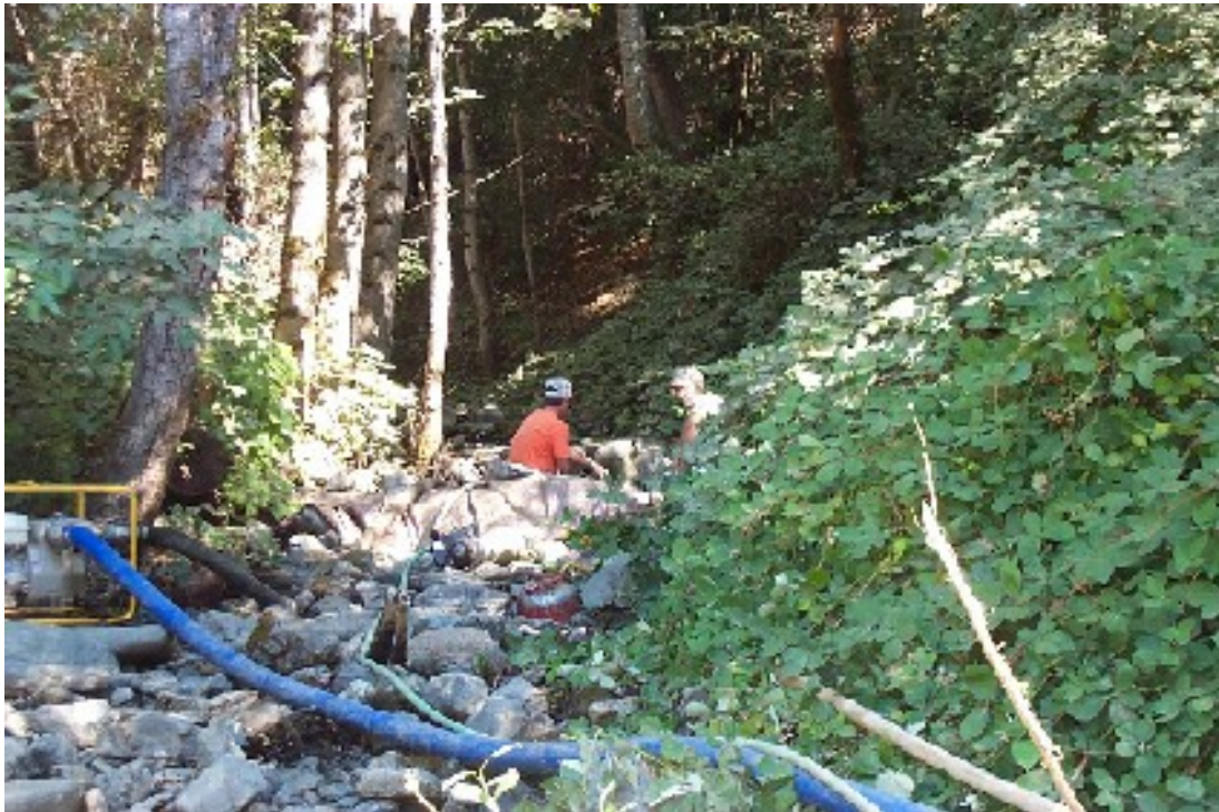
Stream diversion during construction
