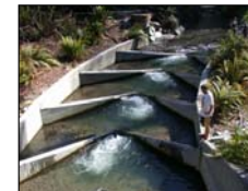
Looking upstream at fishway exit.
