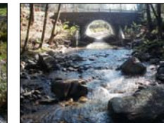
Looking upstream at fishway entrance.
