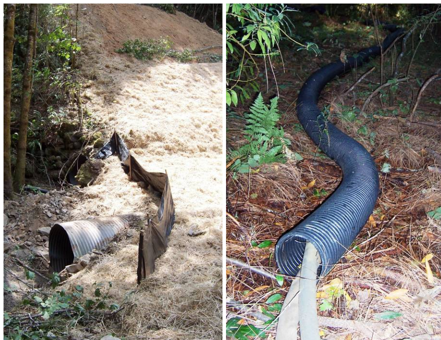
Left - Straw mulch and silt fencing was used during extended shut down periods to prevent erosion and delivery of sediment from the excavation site. Right – use of perforated pipe to distribute turbid discharge across the floodplain.
