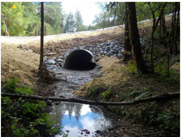
Upper Left Outlet of 5' diameter culvert before project. Upper Right- Inside old culvert showing disconnected segments and rotted bottom. Middle Left- Looking upstream pre-project. Middle Right Fill excavated to culvert depth. Bottom Left- New 14' x 12' (with 3' embedded) arch in place. Bottom Right- 40' deep cut to get new culvert in place.
