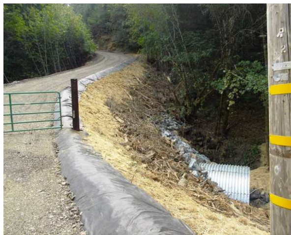
Upper Left- Replacing the road fill. Upper Right- Placing rock slope protection while rebuilding road. Middle Left- Upstream of inlet. Middle Right- Road roughed in. Bottom Left- Road roughed in. Bottom Right- Road in place with only "guard rails" remaining to be installed.
