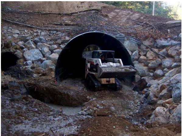
Upper Left- Digging below stream grade to set arch. Upper Right- The creek bed was dewatered and culvert alignment and grade set. Middle Left- Managing the spoils pile. Middle Right- Unloading the arch pieces. Bottom Left- Filling the stream bottom with material. Bottom Right- Streambed in place.
