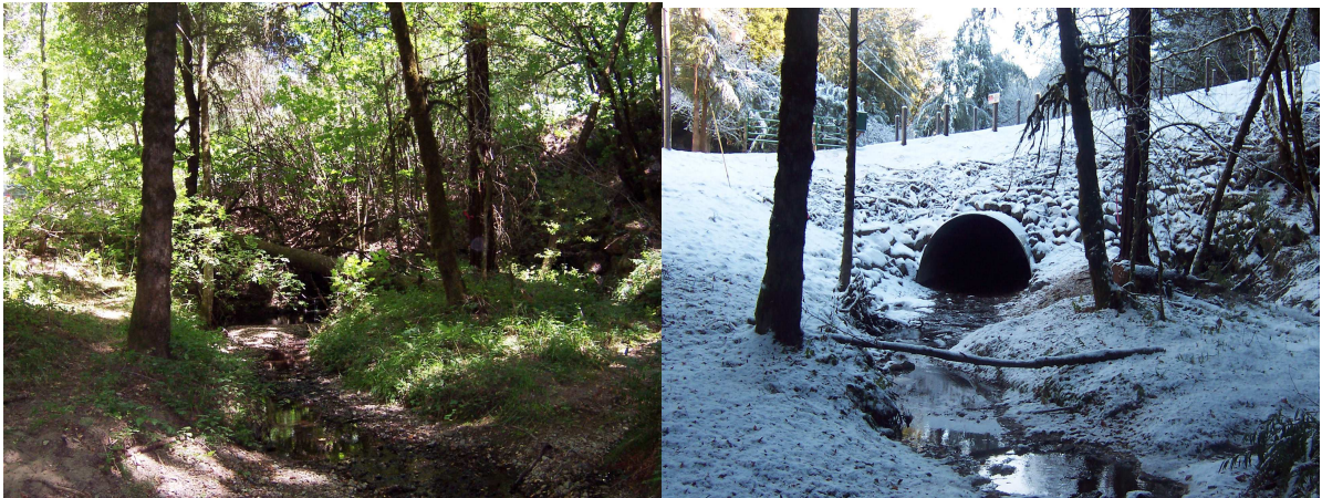
Rhine Driveway Project before with 5' corrugate metal culvert looking upstream (left) and restored channel with 14' wide multi-plate arch culvert (right).
