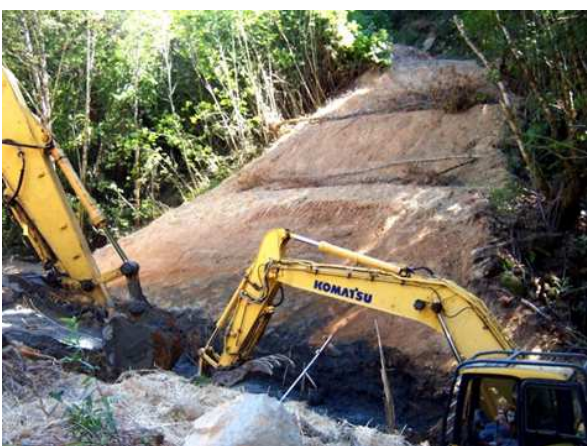
Upper Left Outlet of 5' diameter culvert before project. Upper Right- Inside old culvert showing disconnected segments and rotted bottom. Middle Left- Looking upstream pre-project. Middle Right Fill excavated to culvert depth. Bottom Left- New 14' x 12' (with 3' embedded) arch in place. Bottom Right- 40' deep cut to get new culvert in place.
