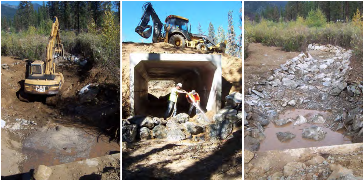
Figures 12 to 16. Upstream channel construction began with cutting excess material and preparing the channel bottom (Left). Jetting fine sand and clay into voids in a grade structure (Middle). Placing the roughened channel bottom, grade structures and apron upstream of the crossing inlet (Right).
