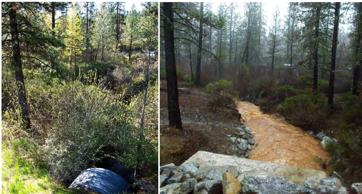
Figure 24-Figure 27. Above (Left) Upstream on December 20 th , 2015 and Above (Right) on January 17 th , 2016 during a ~Q 7 flow. Below Left- Pre-project looking downstream of outlet of 7’ culvert and Right looking downstream during Q 7 flow on January 17 th , 2016 from 12’ x 6’ box culvert.
