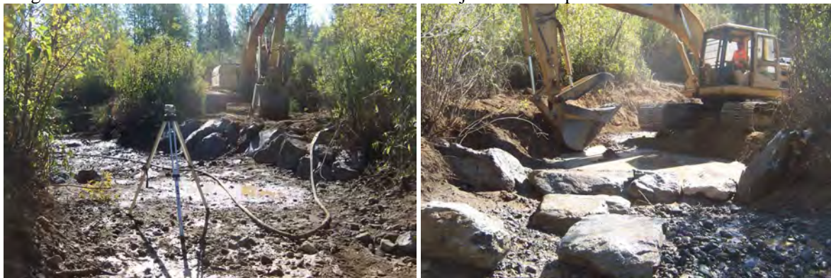
Figures 17 and 18- Channel grade was set with a level and large grade rocks set in the channel and on the banks.
