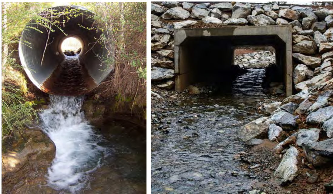
Figures 1 and 2: Pre-project jump and 5% channel gradient in the 7' diameter metal culvert made it impassible to fish migrating upstream. Above left the 12' x 9' box culvert was imbedded 3' and allows for migration on all fish flows.
