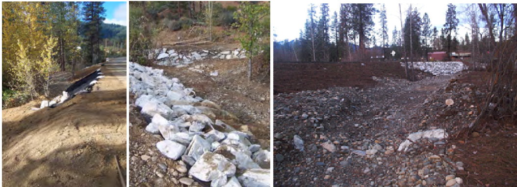
Figure 19 - 21- The overflow channel on the downstream side of the road was designed with larger RSP where the water overtops the road and a return channel to Sidney Gulch.
