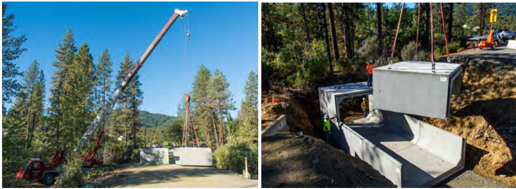
Figures 6 to 11. Box culvert segments being lifted from the road and set in the project site
