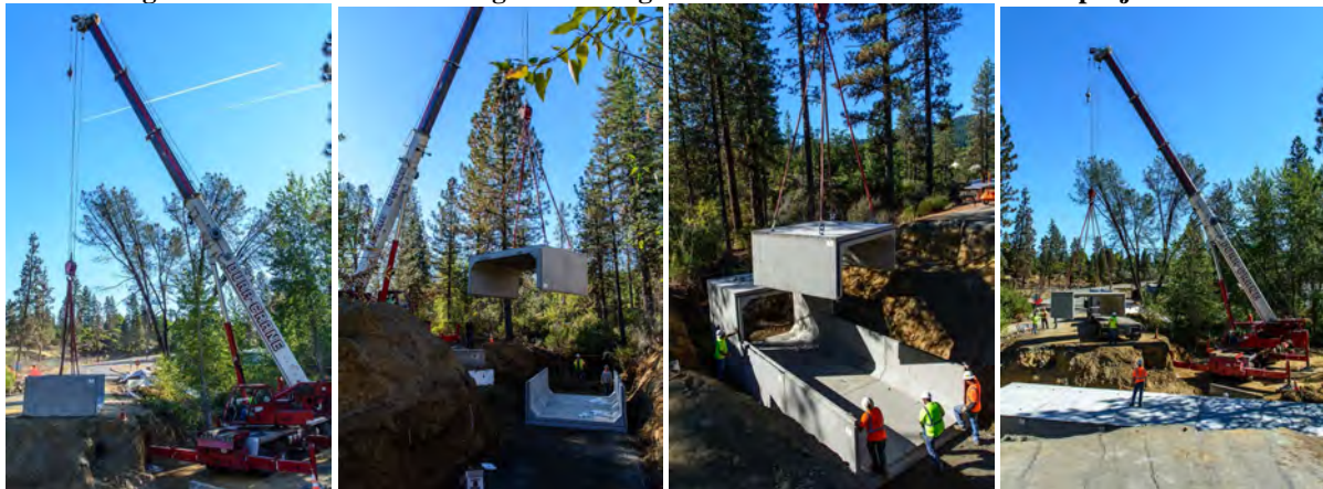
Figures 6 to 11. Box culvert segments being lifted from the road and set in the project site
