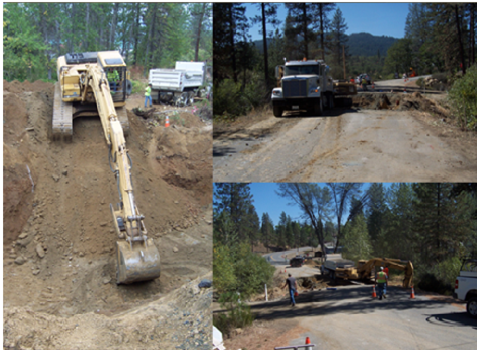
Figures 3-5. Excavating the road fill and preparing the bottom for placement of box culvert segments (Above left). The road excavation (Right)
