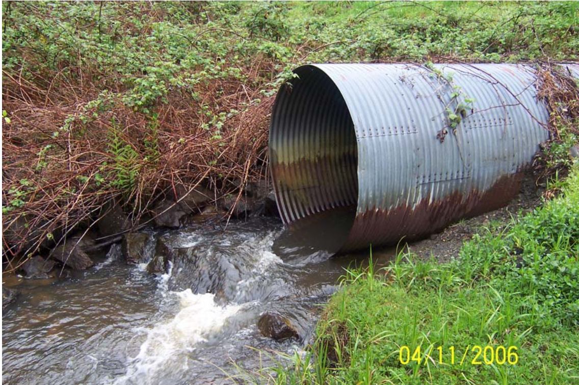
Figure 3 – Migration Barrier Yonkers Creek Outlet
