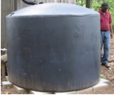
Figure 6. Large polyethylene tanks in various shapes and sizes can be used for storage of water, as long as the material and prior contents were nontoxic. Above ground tanks should be painted black or green.
