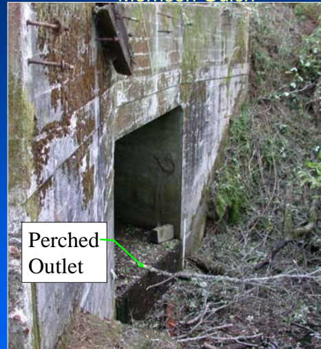
Perched Outlet Channel upstream of culvert replaced with natural regrade
