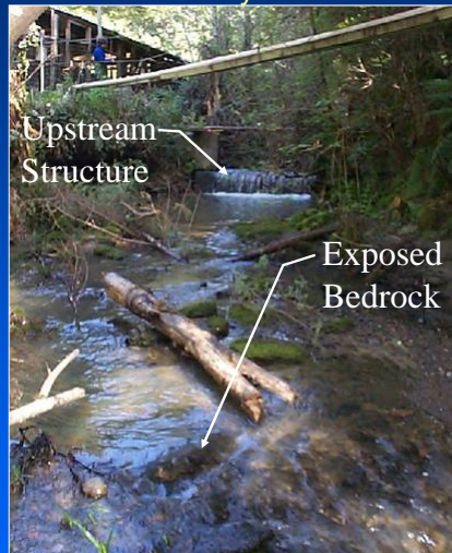
Upstream of perched culvert, prior to removal
