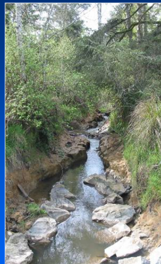
Incised channel upstream of culvert replacement
