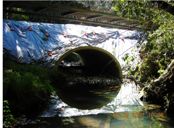
The pictures show a culvert replacement on the Albion River. A silt fence and seeding was used to control erosion (left). Erosion control fabric was installed on the fill slope prior to winter rains (right).
