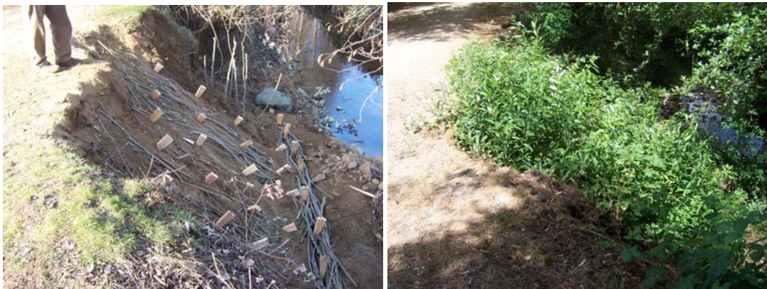
Small scale stream bank stabilization project using bioengineering methods in progress (left) and two years later (right), Sidney Gulch, Trinity County
