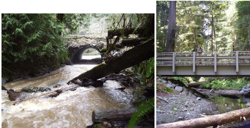
On both public and private lands, many migration barriers have been replaced with “fish friendly” culverts (left, Graham Gulch, Humboldt County) and bridges (right, Del Norte County) thereby restoring access to many miles of stream habitat.
