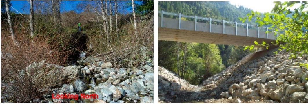
Merrill Creek fish passage barrier (left) was replaced with a bridge and the channel was restored to its natural gradient (right), a project undertaken by Siskiyou County.
