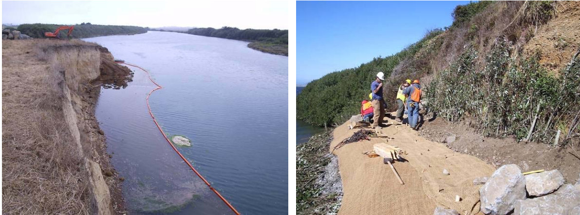
A large bio-engineered bank stabilization project on the Mad River undertaken by Humboldt County Public Works Department
