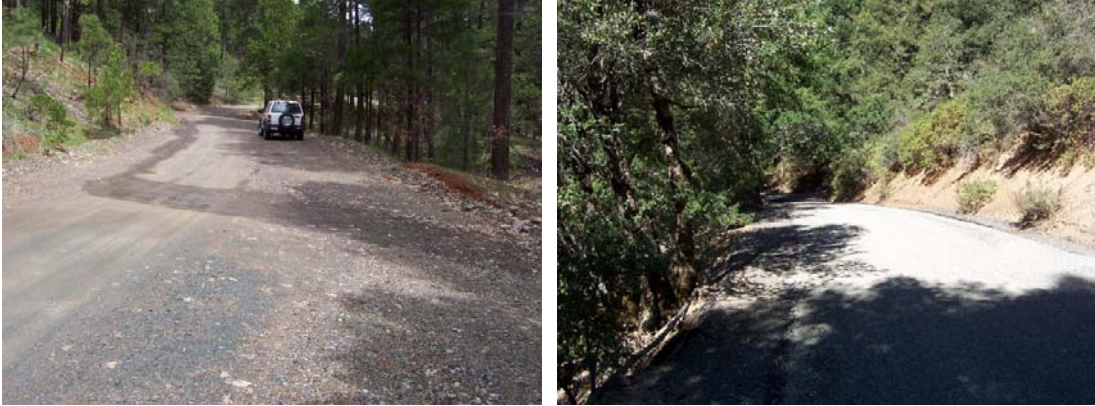
Completed out-sloping and rolling dips on treated low traffic volume county roads (China Gulch on left and Indian Creek Road on right).
