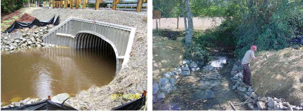
Straw mulch, silt fences and armoring at upgraded stream crossing (top). Erosion control fabric, armoring and willow staking on channel downstream from crossing (bottom).
