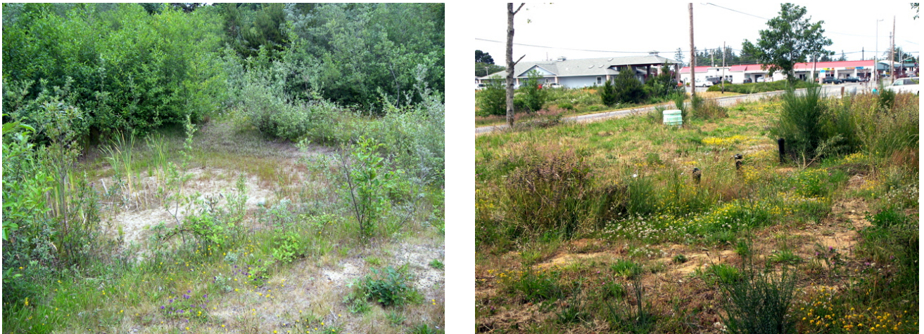
Retention basin serving to store runoff from parking lot (left).
