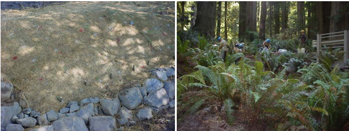
Detail of erosion control and willow staking (left). Re-vegetation with ferns at upgraded stream crossing (right).
