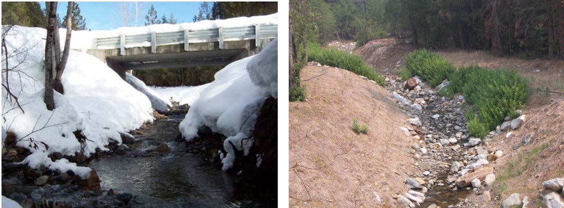
Salmonid migration barrier removal and upslope bioengineered stream bank stabilization and restored channel installed at stream crossing, Little Brown's Creek.
