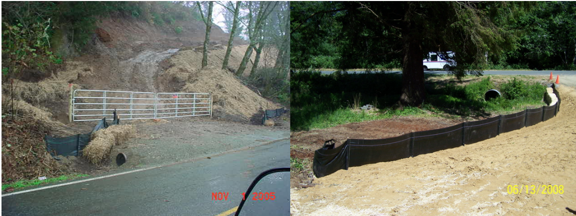
Temporary erosion control measures applied during road construction (left). Silt fence and hay bales installed to prevent sediment delivery to channel (right).
